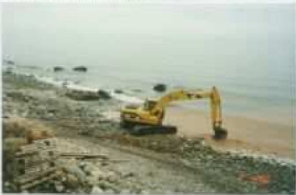
PHOTO 2 SEAL BROOK - DREDGING BASIN
