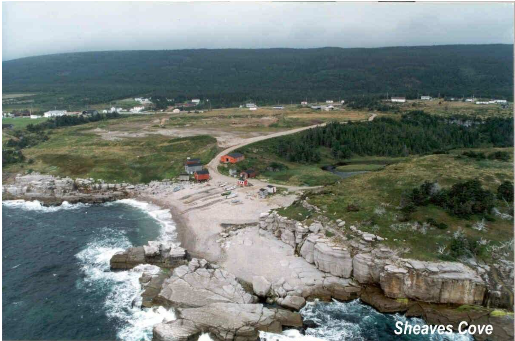
Site Photograph: Aerial View of Sheaves Cove beach levelling site.
