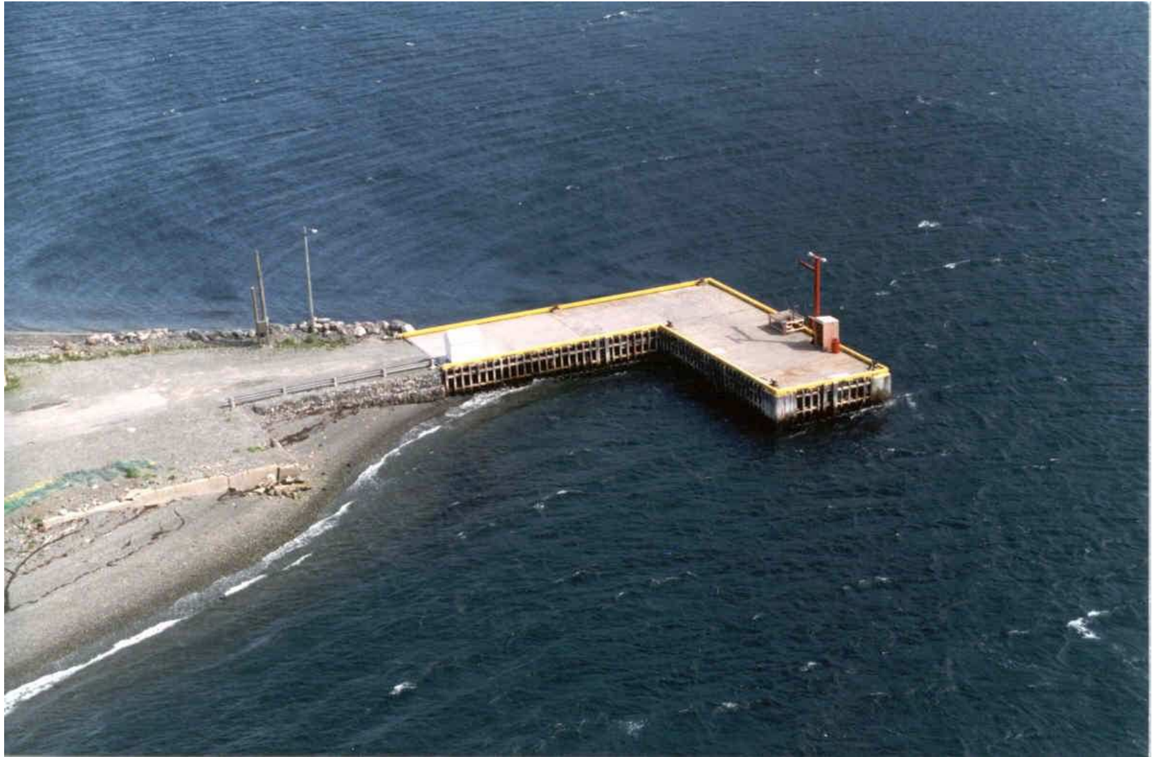
Site Photograph: Aerial view of Lark Harbour dredging site
