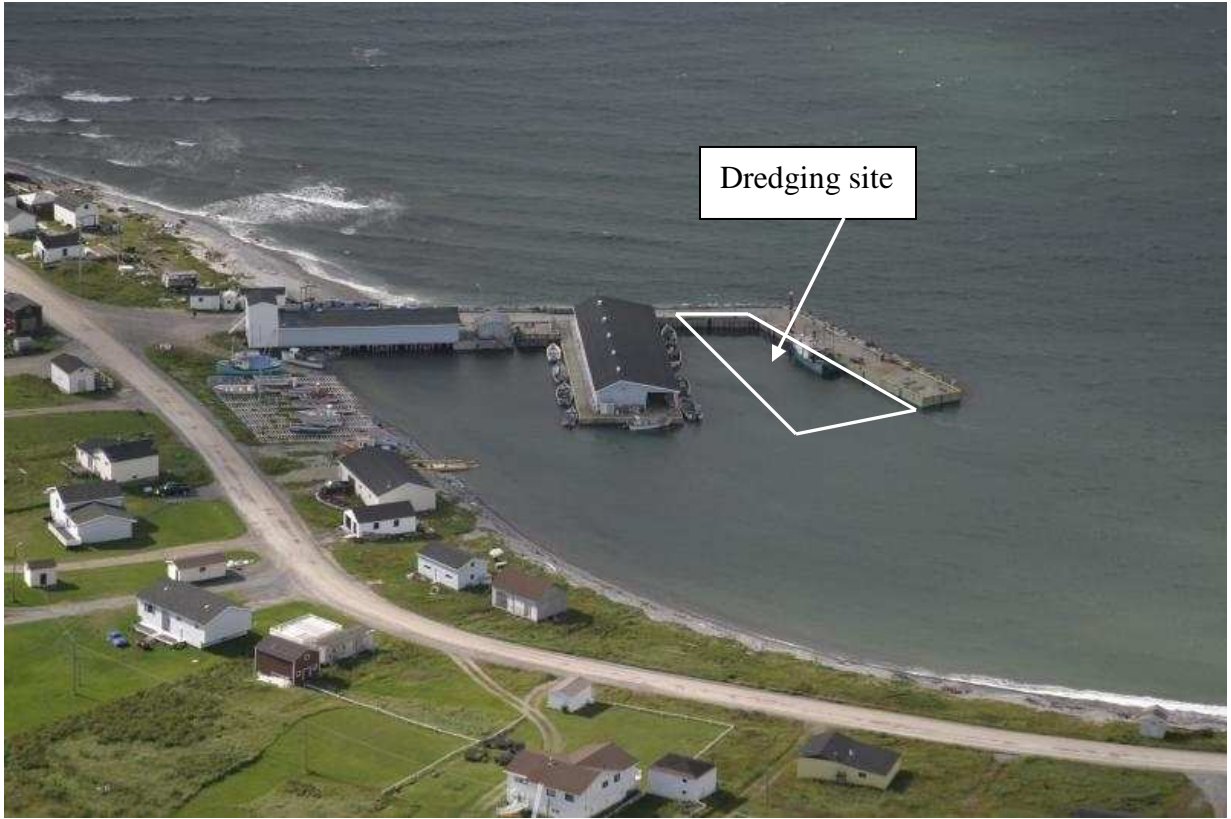
Site photograph: Aerial View of Green Island Cove dredging site.
