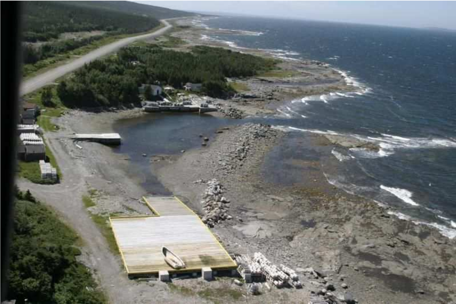
Site Photograph: Aerial View of Josephine's Cove dredging site
