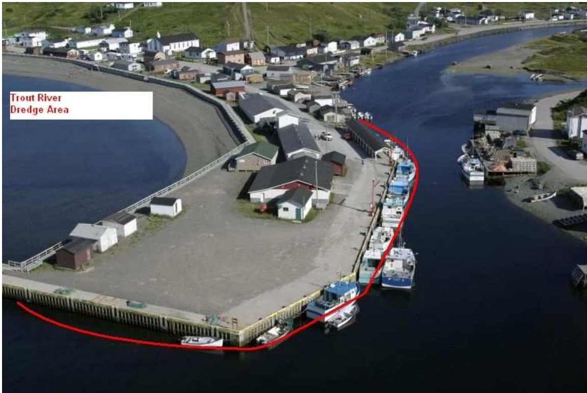
Site photograph: Aerial View of Trout River dredging site.
