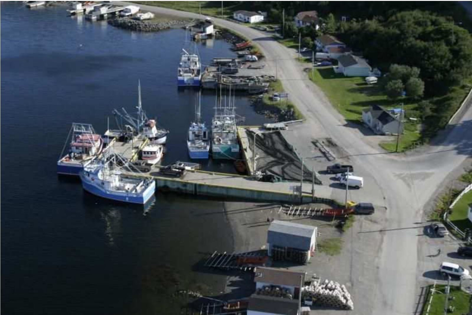
Site Photograph: Aerial View of Frenchman's Cove dredging site.
