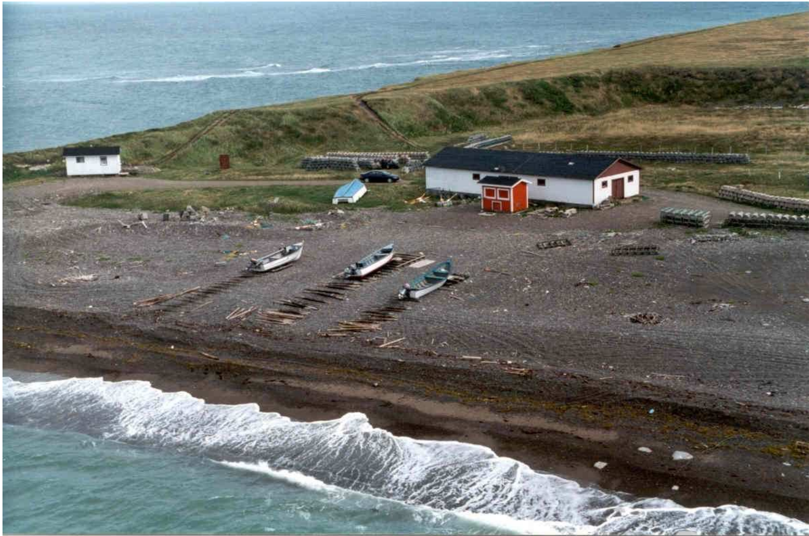
Site Photograph: Aerial View of Three Rock Cove – Penney’s Landing, beach levelling site.
