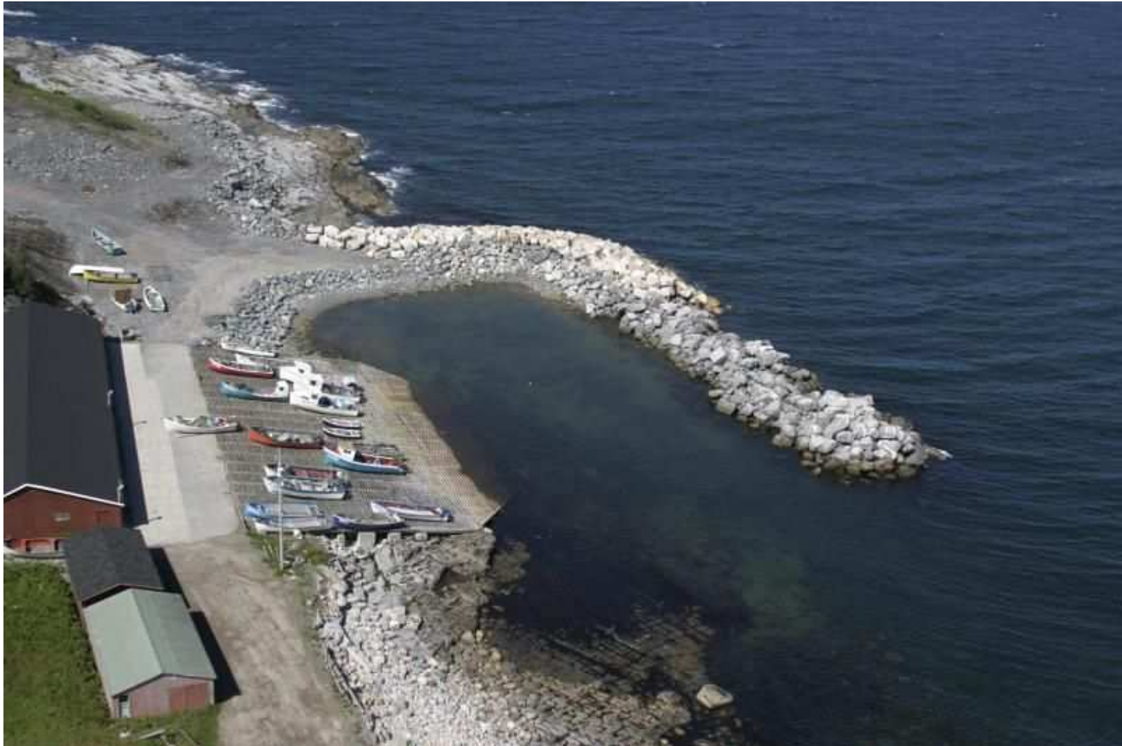
Site Photograph: Aerial View of River of Ponds dredging site.
