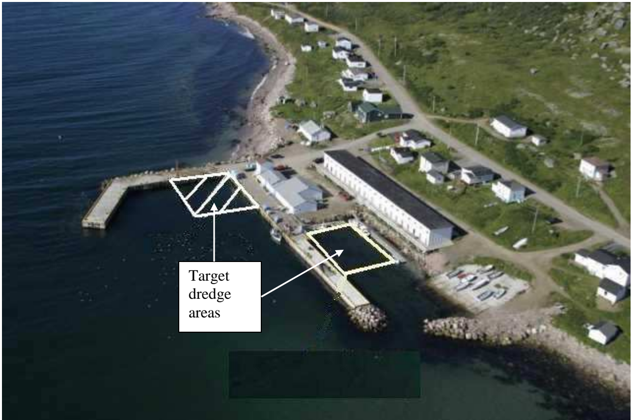
Site Photograph: Aerial View of L'Anse au Clair Cove dredging site.
