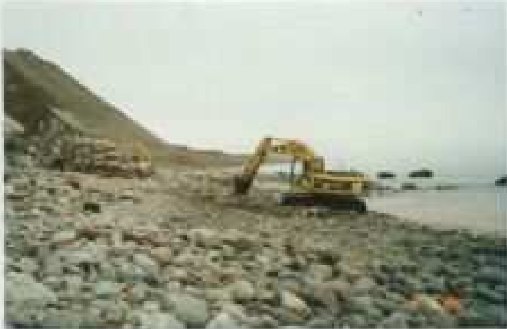
PHOTO 1 SEAL BROOK - BEACH GRADING
