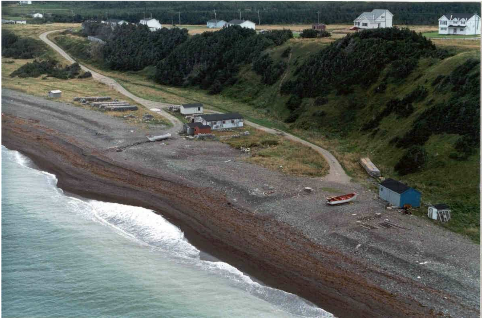
Site Photograph: Aerial View of Three Rock Cove – Collier’s Landing, beach levelling site.
