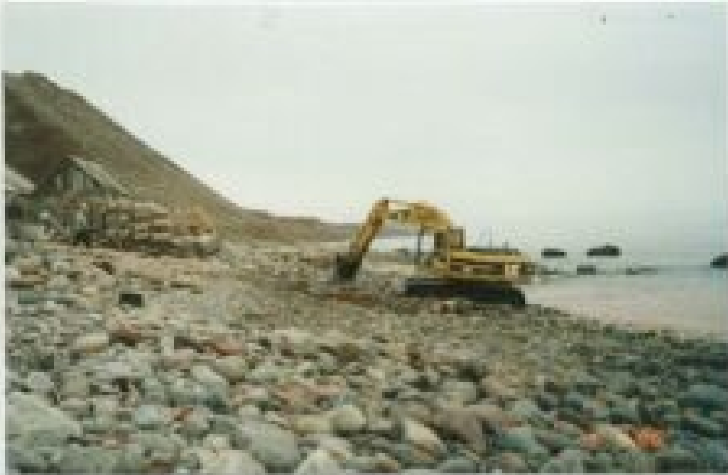
PHOTO 1 - SEAL BROOK - BEACH GRADING
