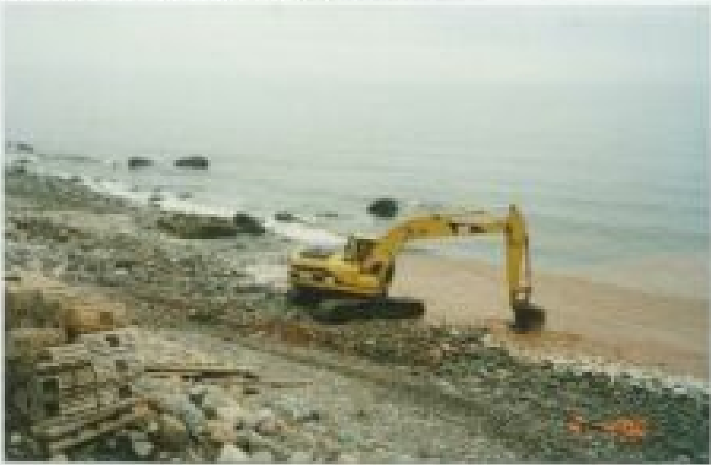
PHOTO 1 - SEAL BROOK - DREDGING BASIN
