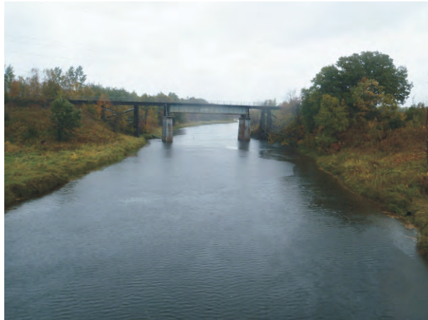
Lower Pinewood River: PIN-18 Facing Upstream
