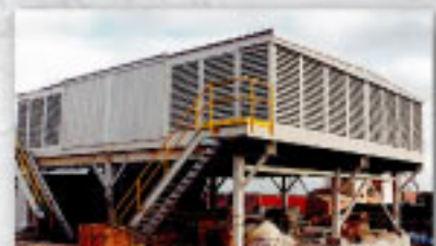
1,000,000 SCFM Direct Fired, Vertical Discharge Mine Air Heater - Natural Gas
