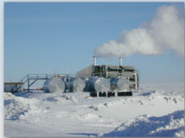
350,000 SCFM Indirect Fired Mine Air Heater - Waste Oil
