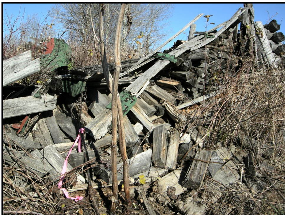
Figure 100. Photograph 267 of the early woodshed.
