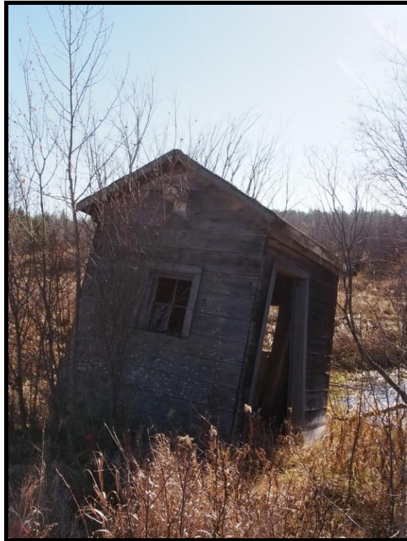
Figure 101. Photograph 769 of the pumphouse by the creek.
