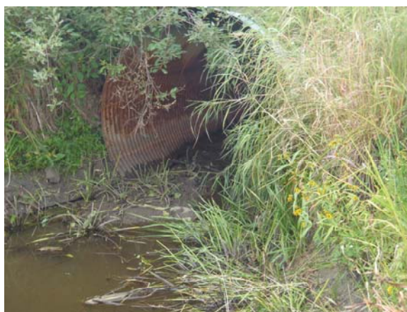
Picture 17: The culvert on the south side of Jones Road.
