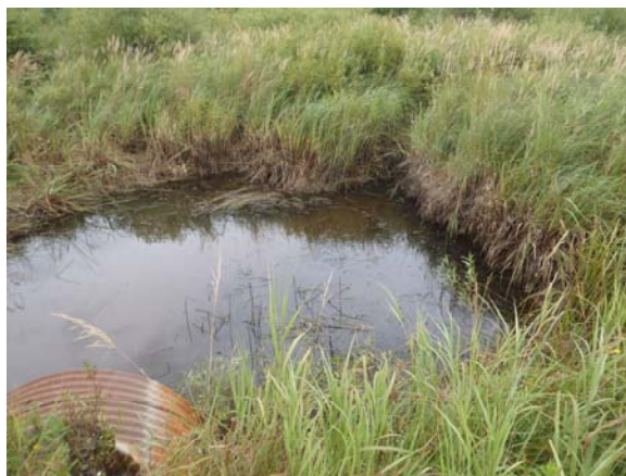
Picture 14: Facing north, culvert inlet basin.
