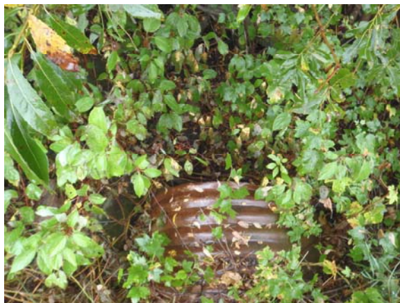
Picture 22: Creek outlet at culvert on north side of creek crossing.
