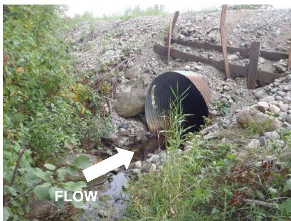
Picture 6: Culvert inlet on east side of Clark road.
