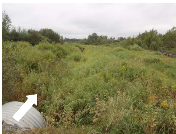
Picture 42: Outlet of culvert on west side of the road.
