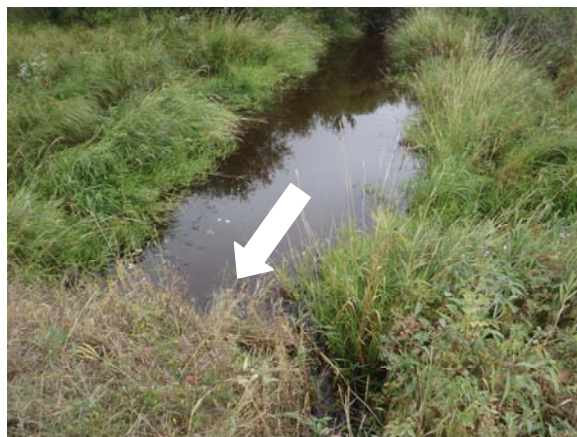
Picture 35: Facing upstream standing on wood box culvert.
