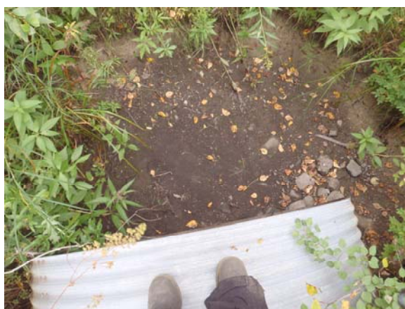
Picture 20: Culvert inlet on the south side of the road.
