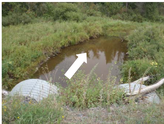
Picture 37: Culvert outlet on west side of the road.
