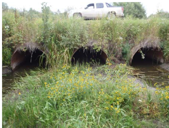
Picture 44: Culverts outlets on the south side of the road.
