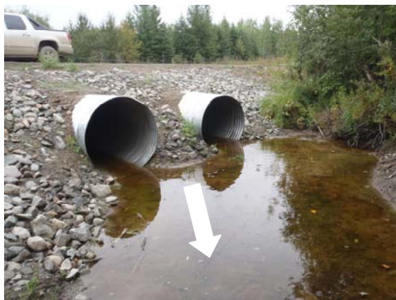
Picture 47: Culvert on south side of road, facing north.
