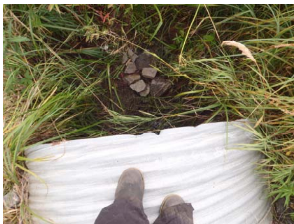
Picture 15: One of three culverts on the south side of Highway 600.
