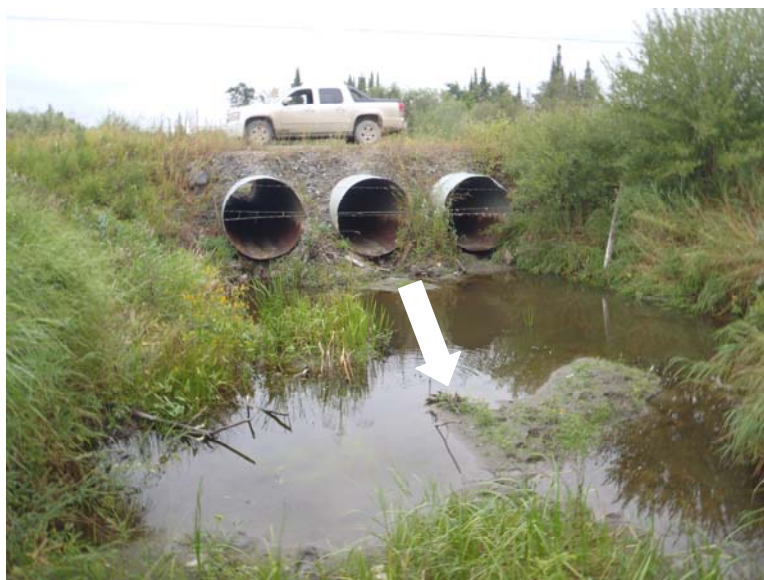
Picture 46: Culvert outlet on the south side of the road.
