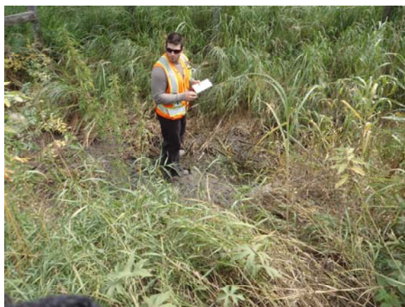
Picture 11: East side of Roen Road, culvert inlet dry.
