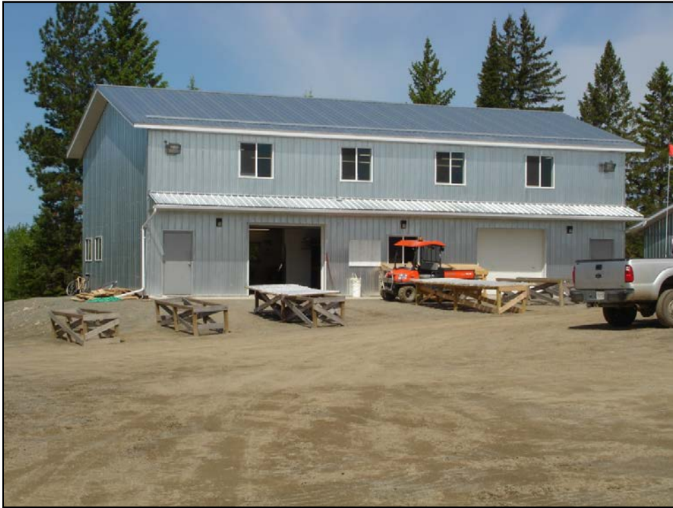
Plate 1: Rainy River Project (RRP) core processing facility
