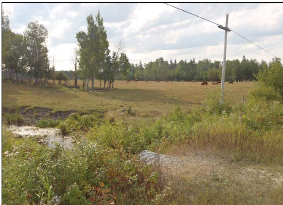
Plate 28: Pinewood River upstream location culvert crossing (August 2011)
