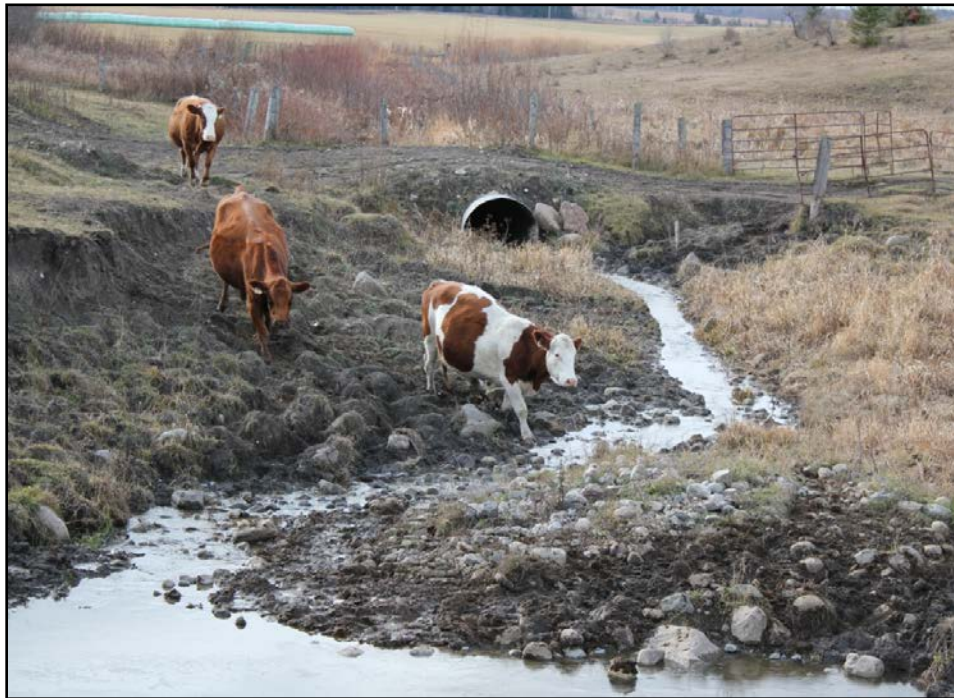
Plate 27: Clark Creek culvert crossing at Clark Road, midstream section (November 2011)
