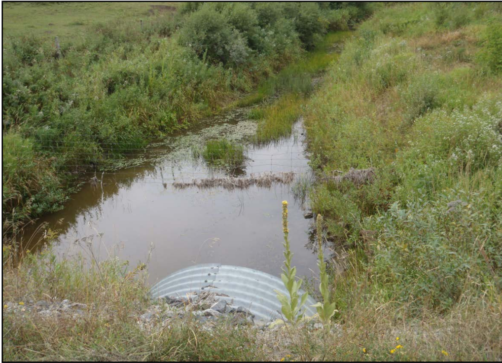
Plate 29: Pinewood River upstream location culvert crossing (August 2011)
