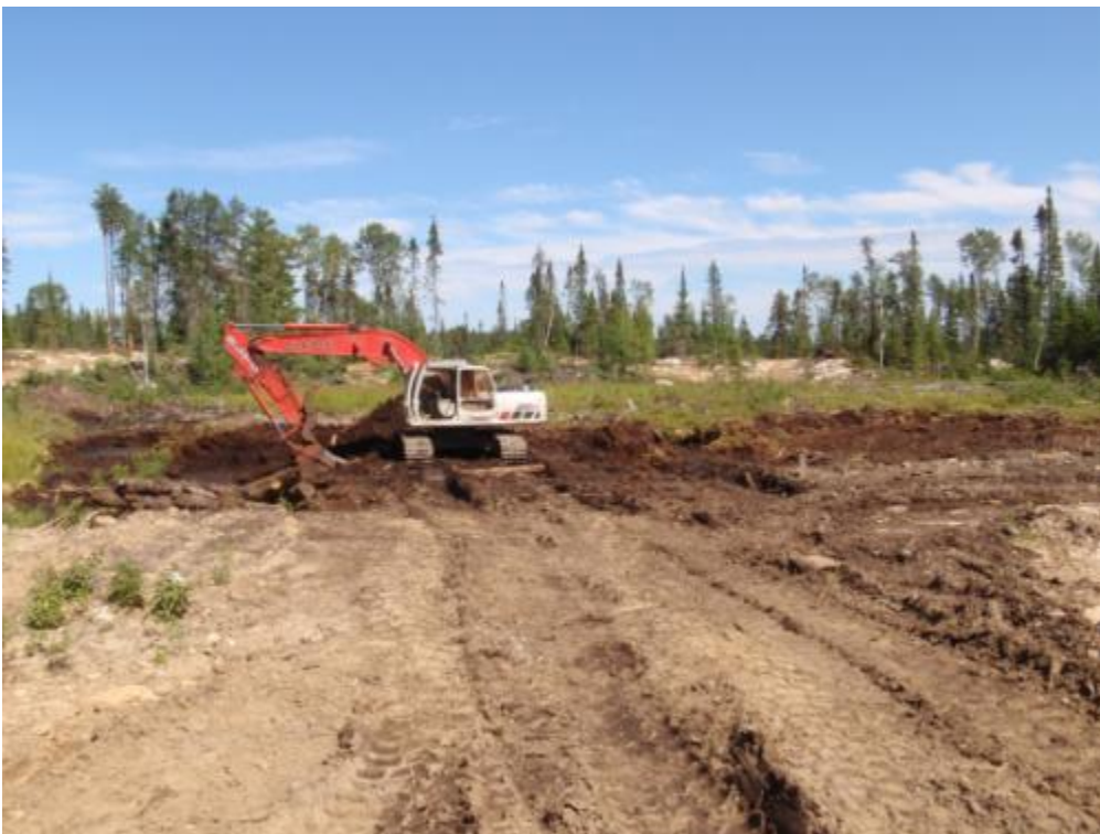
Plate 16: Photo 041, Waypoint P34, backfilling wetlands, facing southeast
