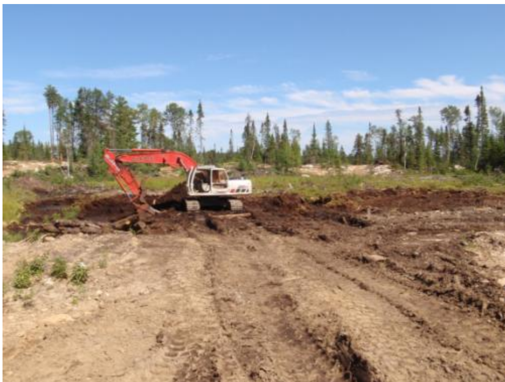
Plate 16: Photo 041, Waypoint P34, backfilling wetlands, facing southeast
