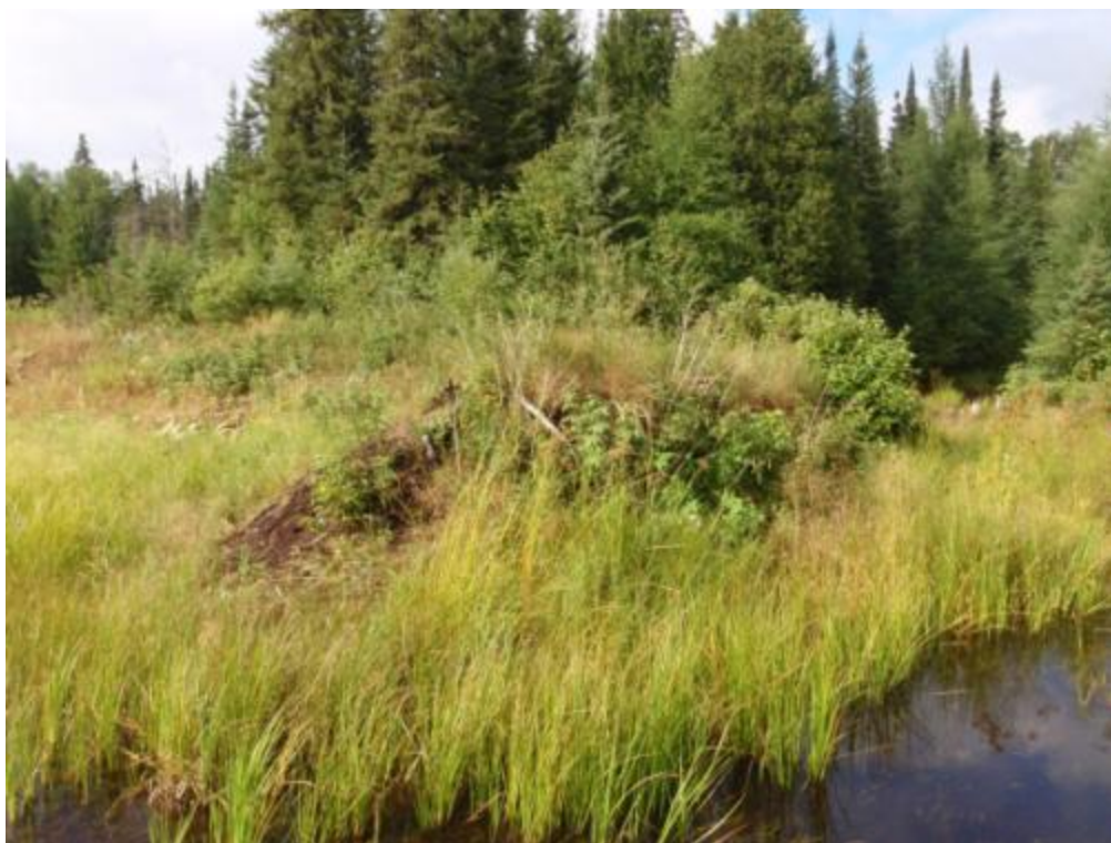
Plate 54: Photo 277, Waypoint k97, Hammond Gold Reef Mine reservoir earth dam, facing east
