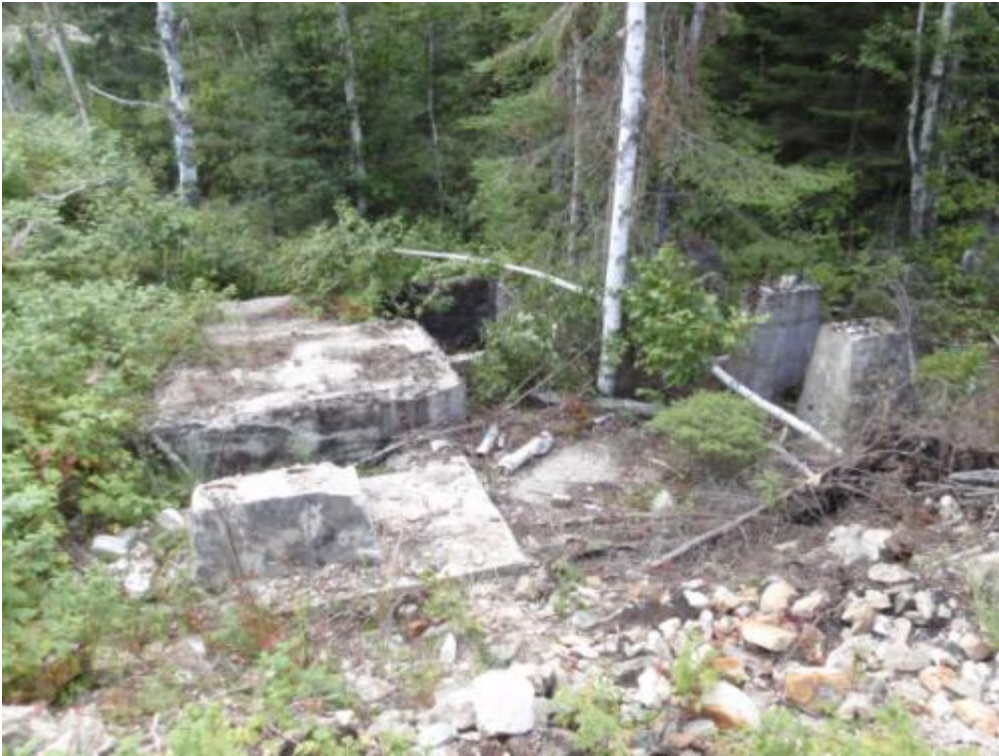
Plate 57: Photo 268, Waypoint 'building', cement foundations, facing southeast
