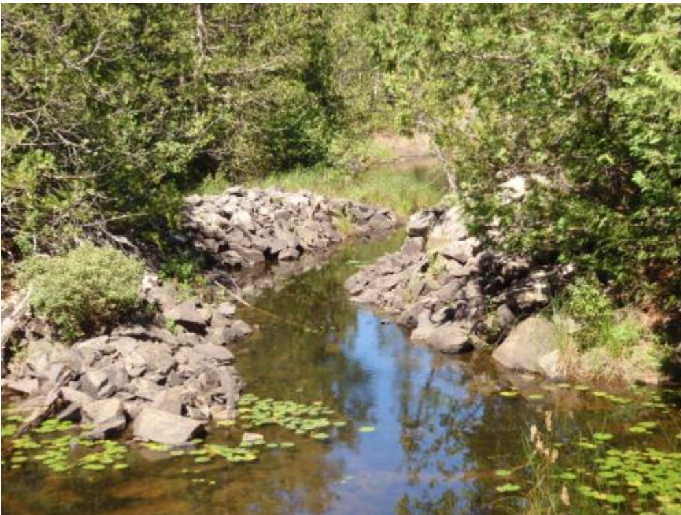
Plate 44: Photo 542, Waypoint 209, modified stone channel, facing west
