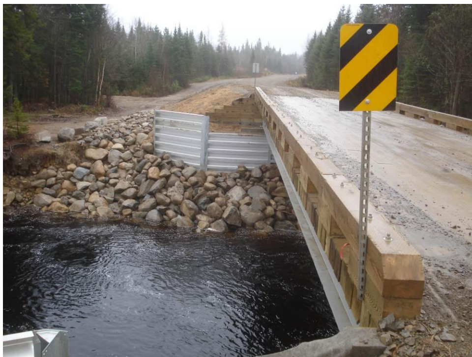
Photo 8.15.3 New single-span, single-lane bridge at Nashwaak River.
