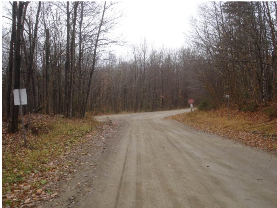
Photo 8.15.2 Fire Road, near the intersection with Napadogan Road, looking eastward.
