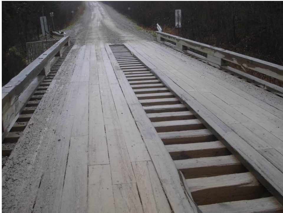
Photo 8.15.4 Single-span, single-lane bridge at Keswick River.
