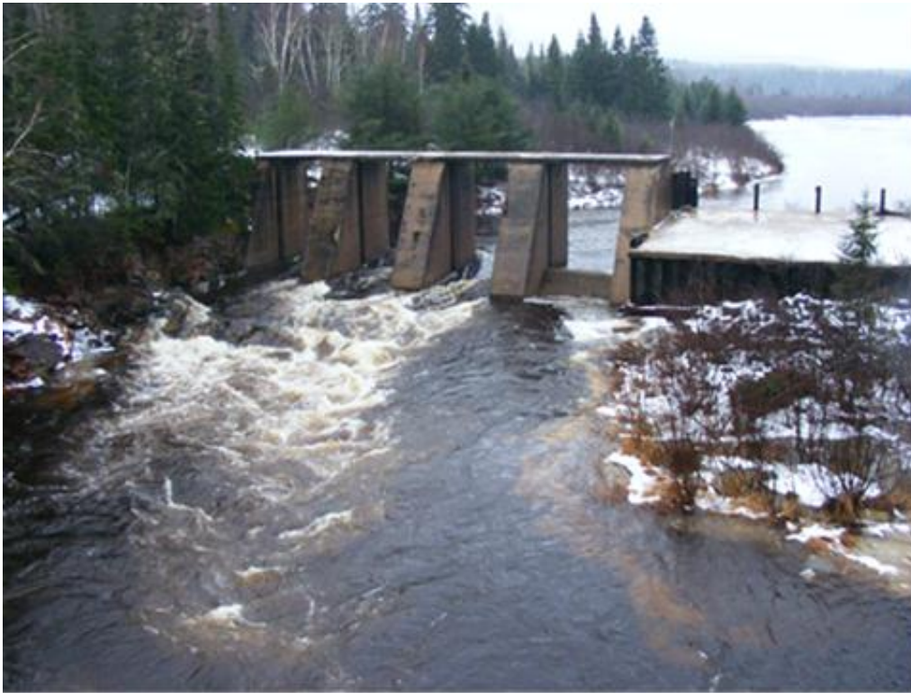
Photo 1: Lower Lake Dam
