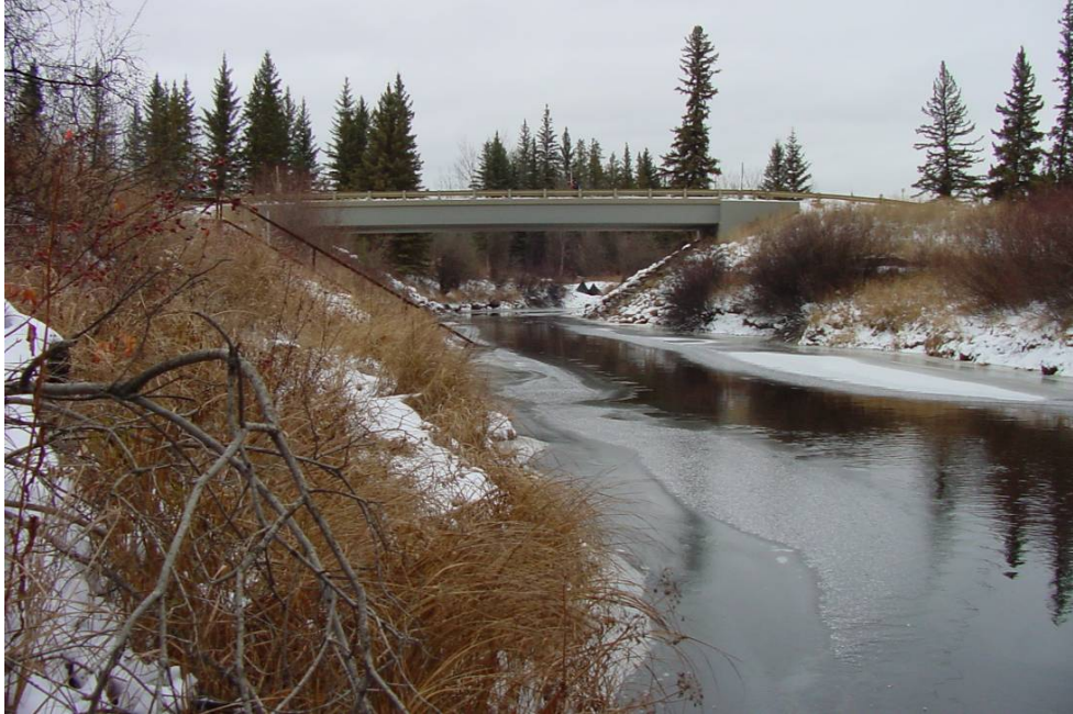
View of HME 4.2 from downstream of the Muskeg River bridge
