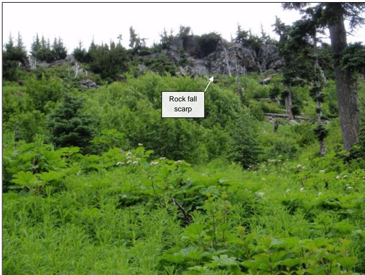
Photograph 16 Treaty Creek Access Road – Looking upslope (north) from Km 26+000 towards an exposed rock bluff with rock fall potential approximately 150 m to 200 m upslope from road alignment. The slope angle to the base of the rock scarp is 33 degrees. Vegetation is dense and well established (>20 years old) suggesting the slope is less active.
