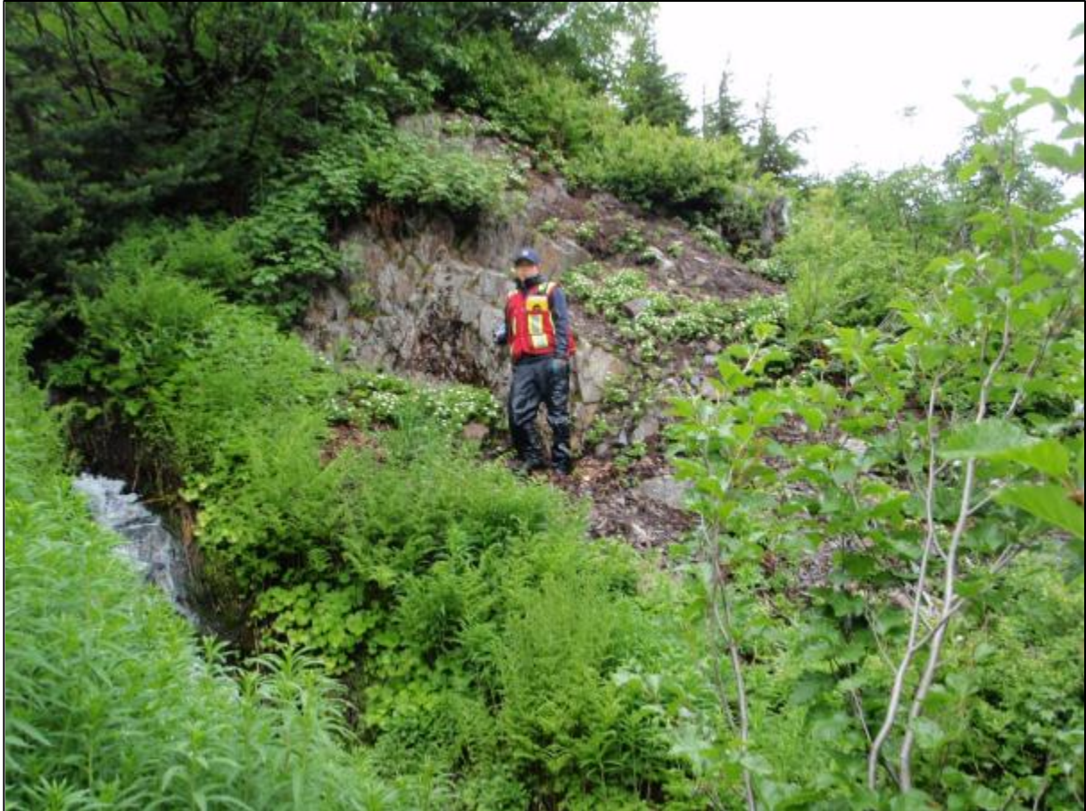
Photograph 17 Treaty Creek Access Road – Looking downchain (east) from left river bank approximately 7 m upslope of Km 26+200 towards an exposure of slightly weathered (W2), weak to medium strong (R2 to R3), sandstone and siltstone.
