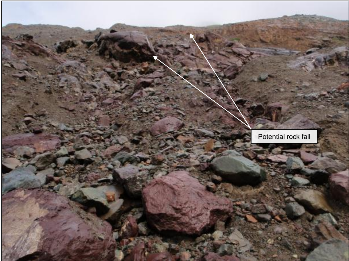
Photograph 31 Tunnel Adit & Tunnel Adit Spur Access Roads – Looking upslope (north) from the Tunnel Adit at Km 2+200 towards rock fall hazards upslope (boulders up to 3 m diameter).
