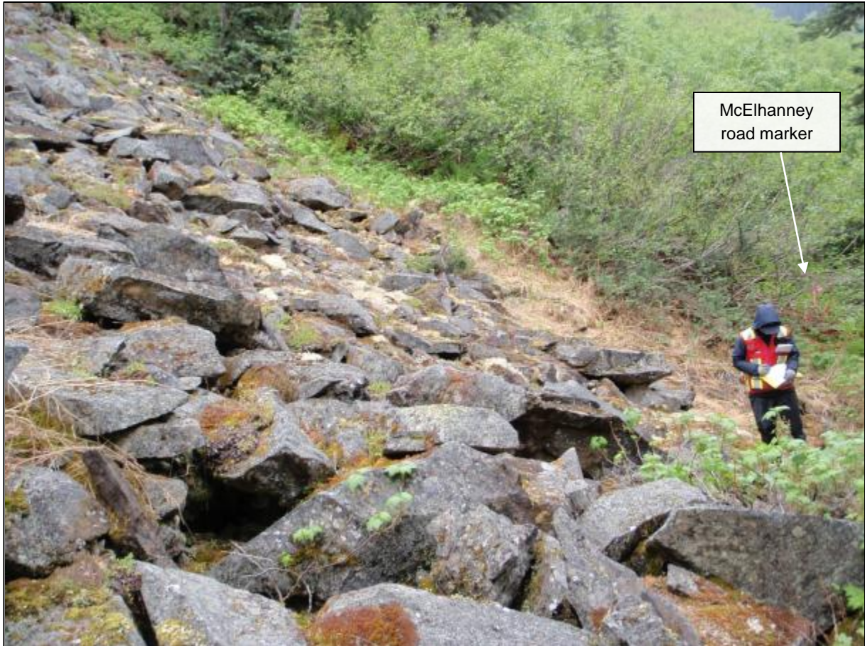
Photograph 11 Treaty Creek Access Road – Looking downchain (east) towards Km 25+420 where the road traverses below a talus slope. Moss covered angular boulders between 1 m and 2 m diameter.
