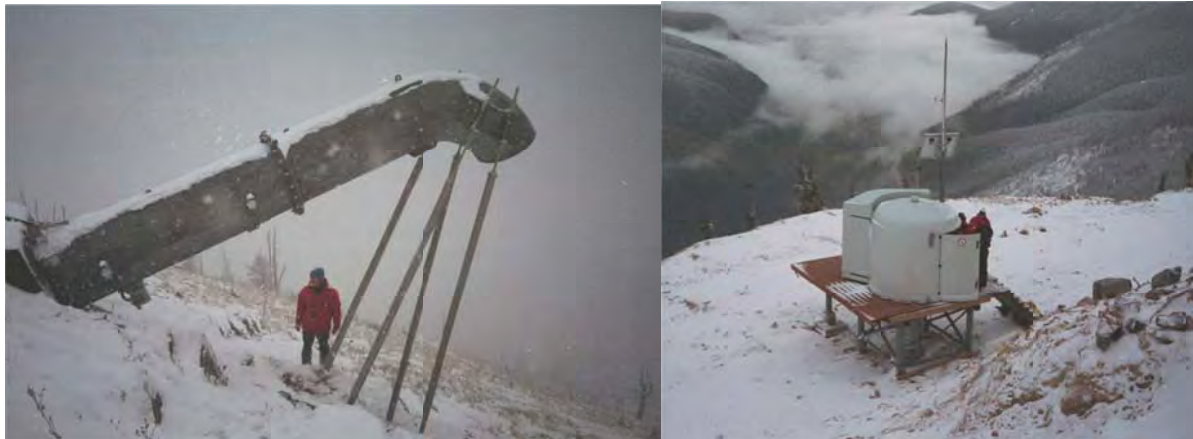
Figure 3-1 – Gas exploder and control shelter
