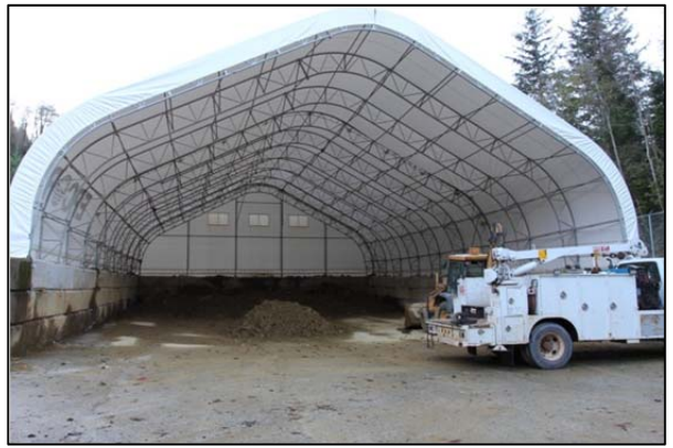
Front View of Sludge Storage Building at Britannia
