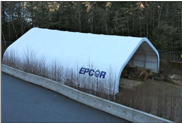
Sludge Storage Building at Britannia
