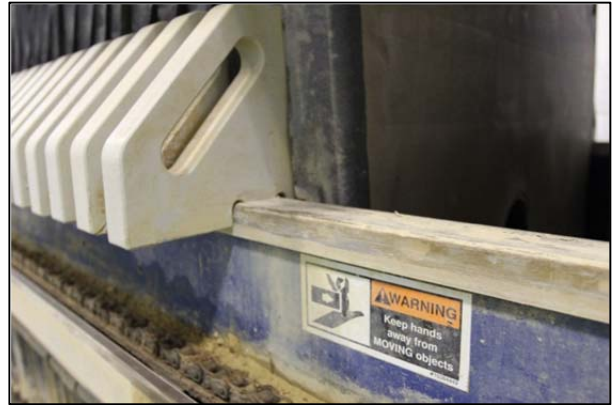
Close-up Filter Press Plate Hangers
