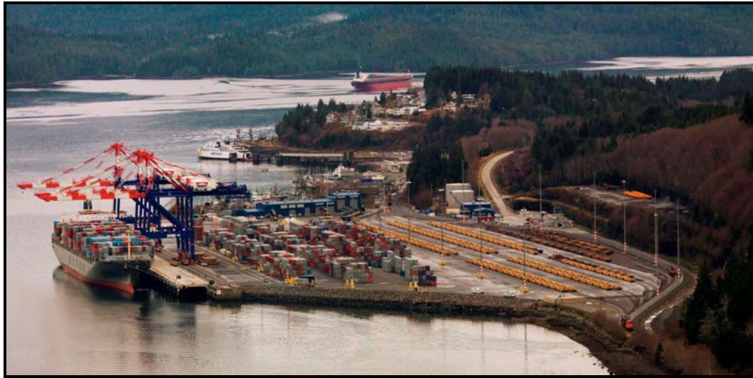
Figure 3.1 Fairview Terminal, Prince Rupert
