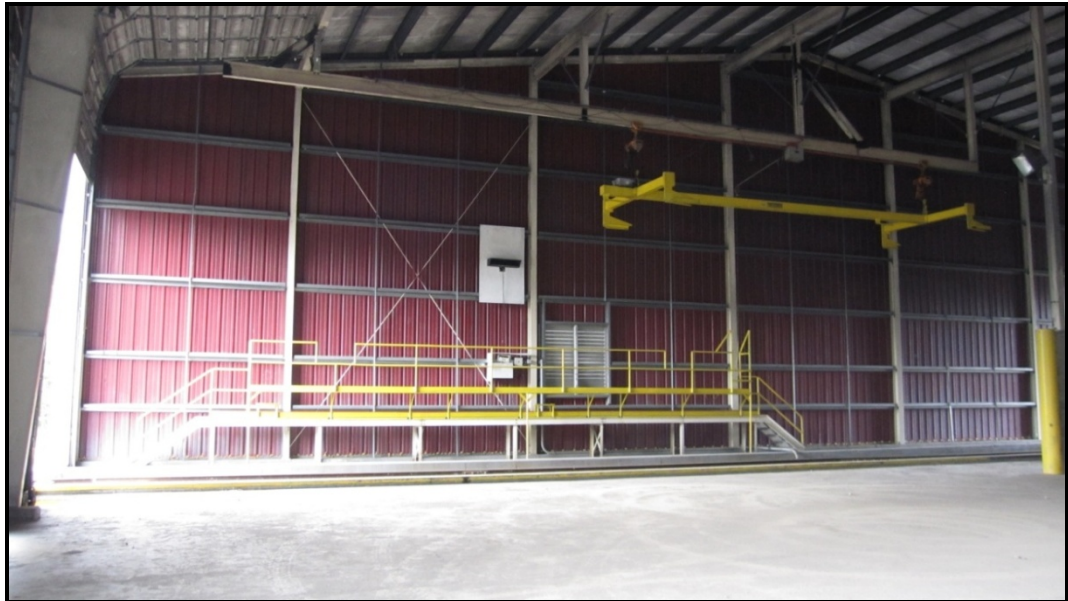
Figure 2.6 Kitwanga Facility Interior – Overhead Crane
