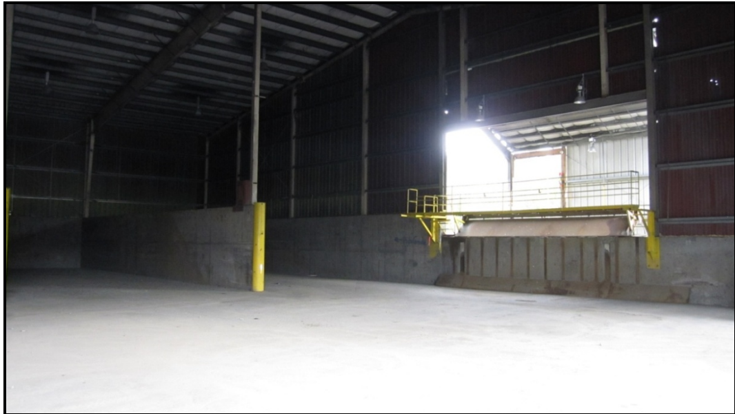
Figure 2.8 Kitwanga Facility Interior – Truck Dump Area
