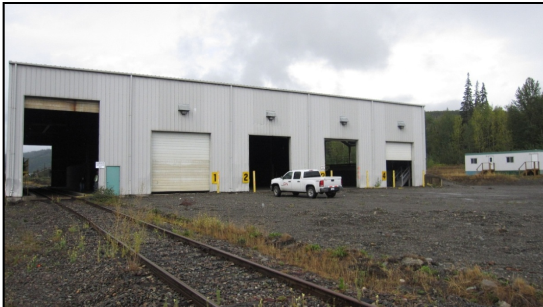
Figure 2.5 Kitwanga Facility Exterior – Rail Access
