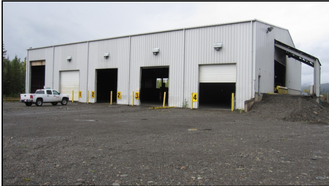
Figure 2.4 Kitwanga Facility Exterior – Truck Bay and Ramp
