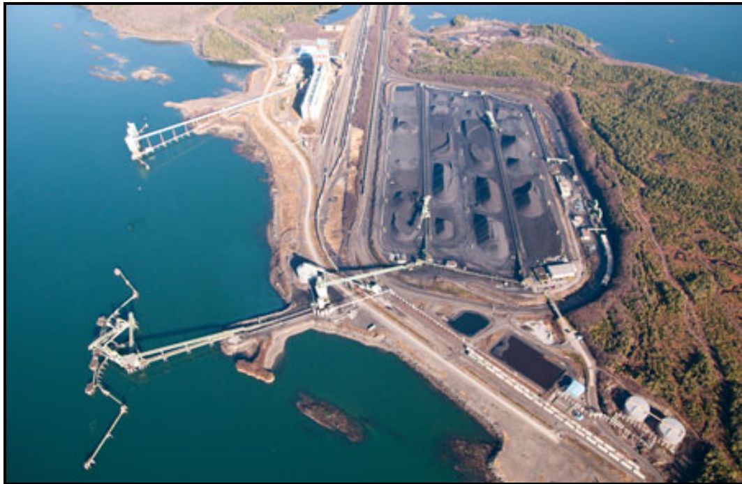
Figure 2.9 RTI Facilities – Aerial Photograph
