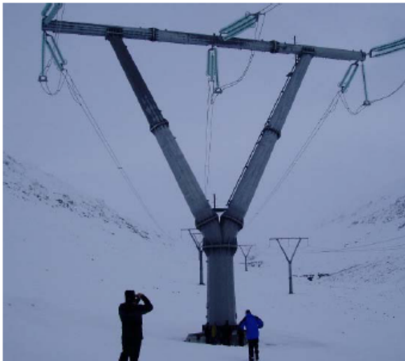
Figure 8.2 - 3 Single Pole Structure On Foundation (Iceland)
