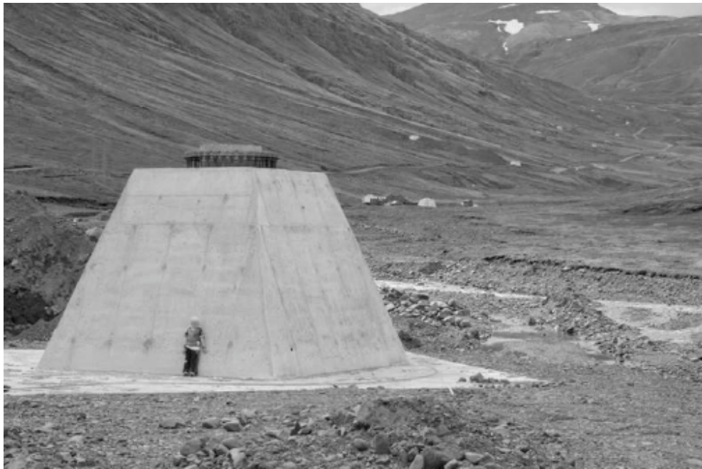
Figure 8.2 - 3 Single Pole Structure On Foundation (Iceland)
