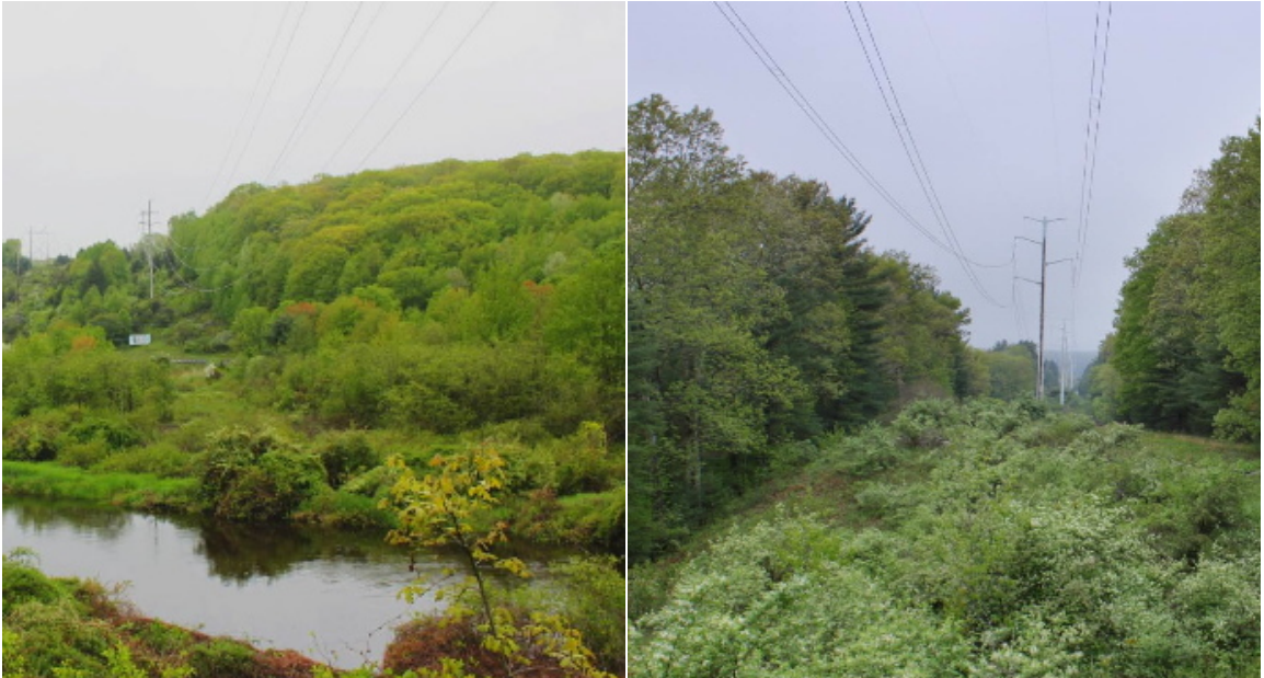
Figure 2.12-1 Examples of ROW Minimal Clearing
