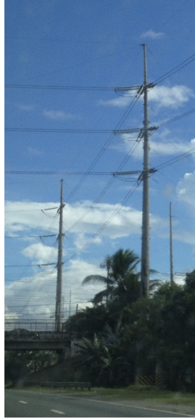
90 Degree Deviation Structures
