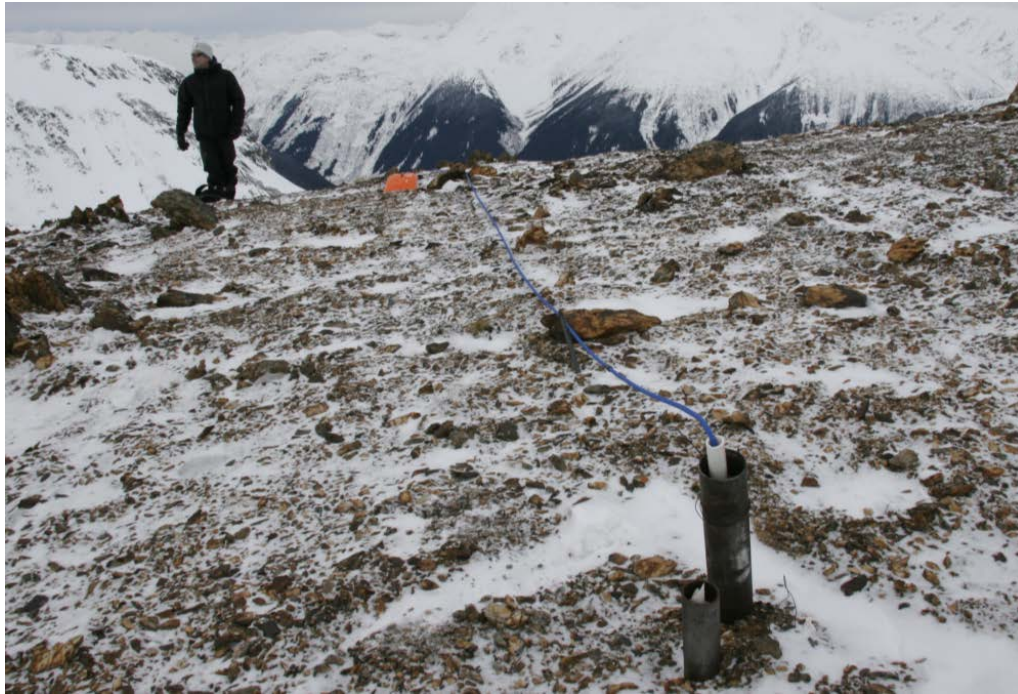
Photo 5: Damaged borehole cover for borehole K-10-07. Little snow cover indicates that high winds are most likely the cause for the damage.
