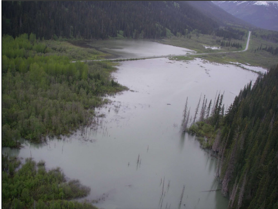
Plate 5.2-1. Flooded Snowbank Creek area around the south culvert.
