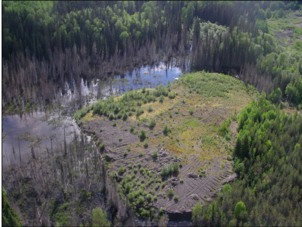
Plate 5.2-4. Load-out area at Van Dyke Camp infilling a large swamp open water complex.
