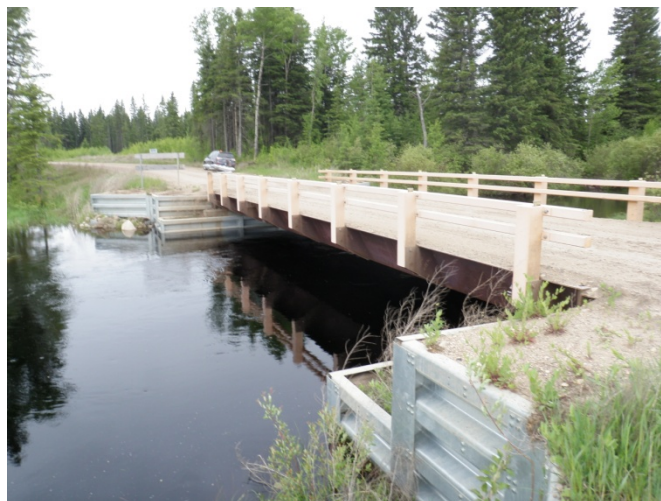
Photograph No. 2 – Bridge Elevation
