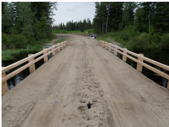
Photograph No. 1 – Centreline of Existing Bridge
