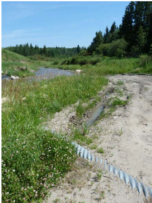
Photo 32. Point B on Figure 6.3.1-3 on Peonan Creek at the road crossing.
