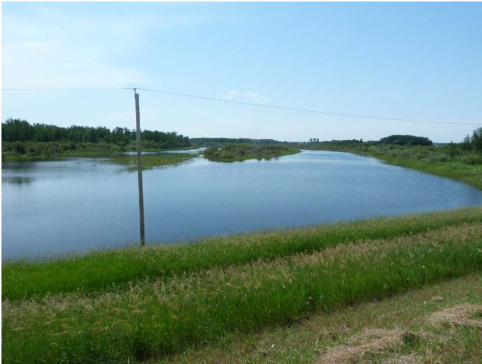
Photo 27. Looking south from the highway at Muskoday bridge (approximately 465780E, 5881635N).
