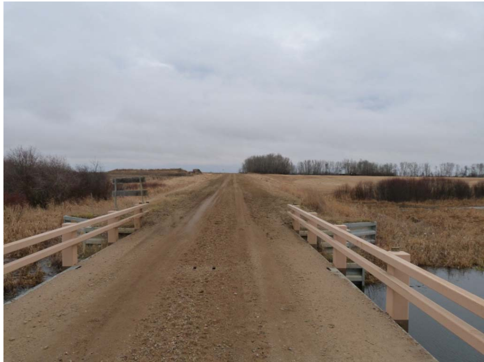
Photo 8. White Fox River crossing looking north, November 2010.
