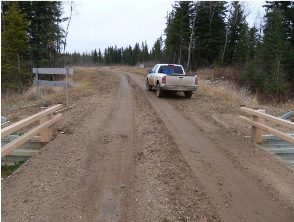
Photo 9. White Fox River crossing looking south, November 2010.
