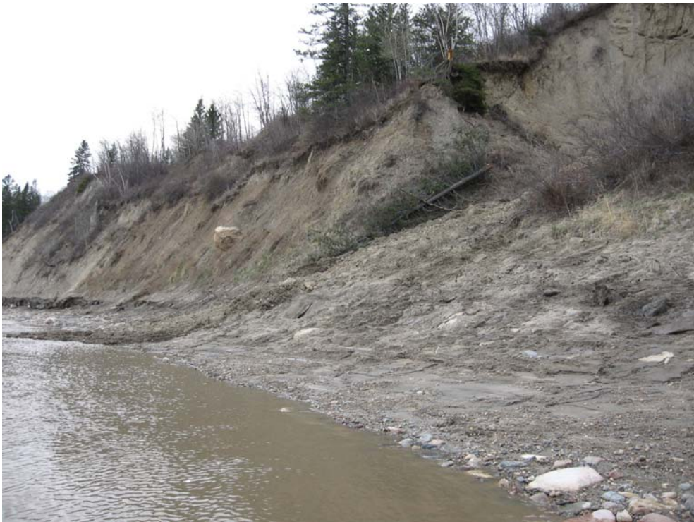
Photo 12. SKR at West Perimeter Ravine representative of HS1.
