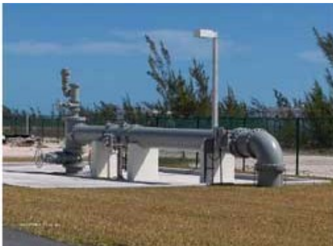
Typical injection well wellhead
