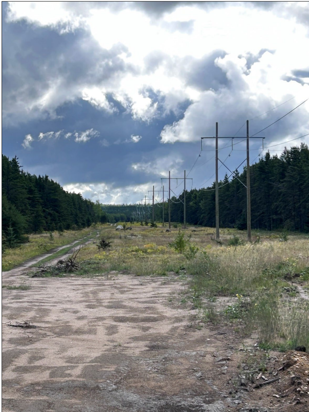
Figure 5.1-3: Existing Regional E2R Transmission Line
