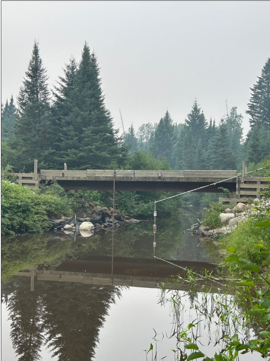
Figure 5.1-2: Existing Bridge over Dixie Creek
