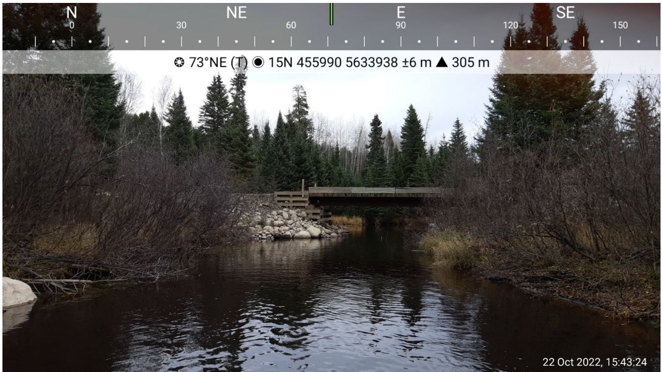
Photo 3. DC-02 – Facing downstream. Oct 22, 2022.
