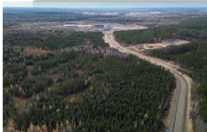
Chukuni Pipeline into AEX site – October 25, 2025
