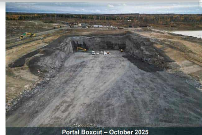
Portal Boxcut – October 2025
