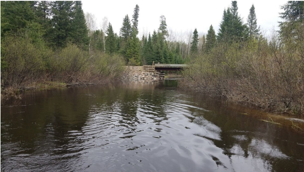
Photo 21: Dixie Creek Bridge, May 2022
