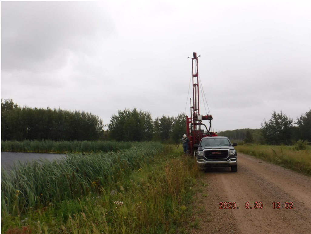
Photograph 3: Looking southeast towards BH20-B01 (existing berms)
