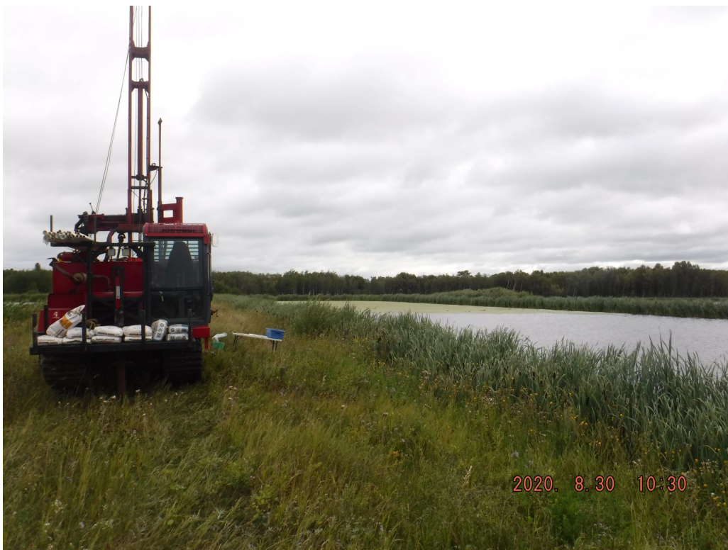
Photograph 4: Looking northeast towards BH20-B10 (existing berms)
