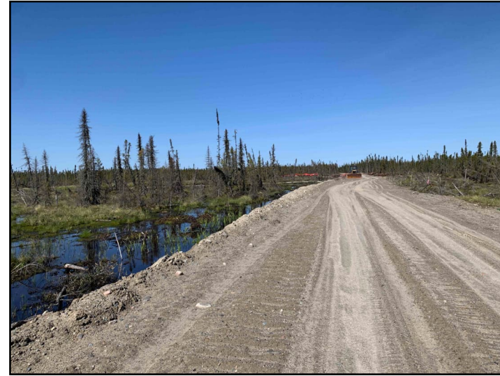
Gravel road through wetland, May 2023
