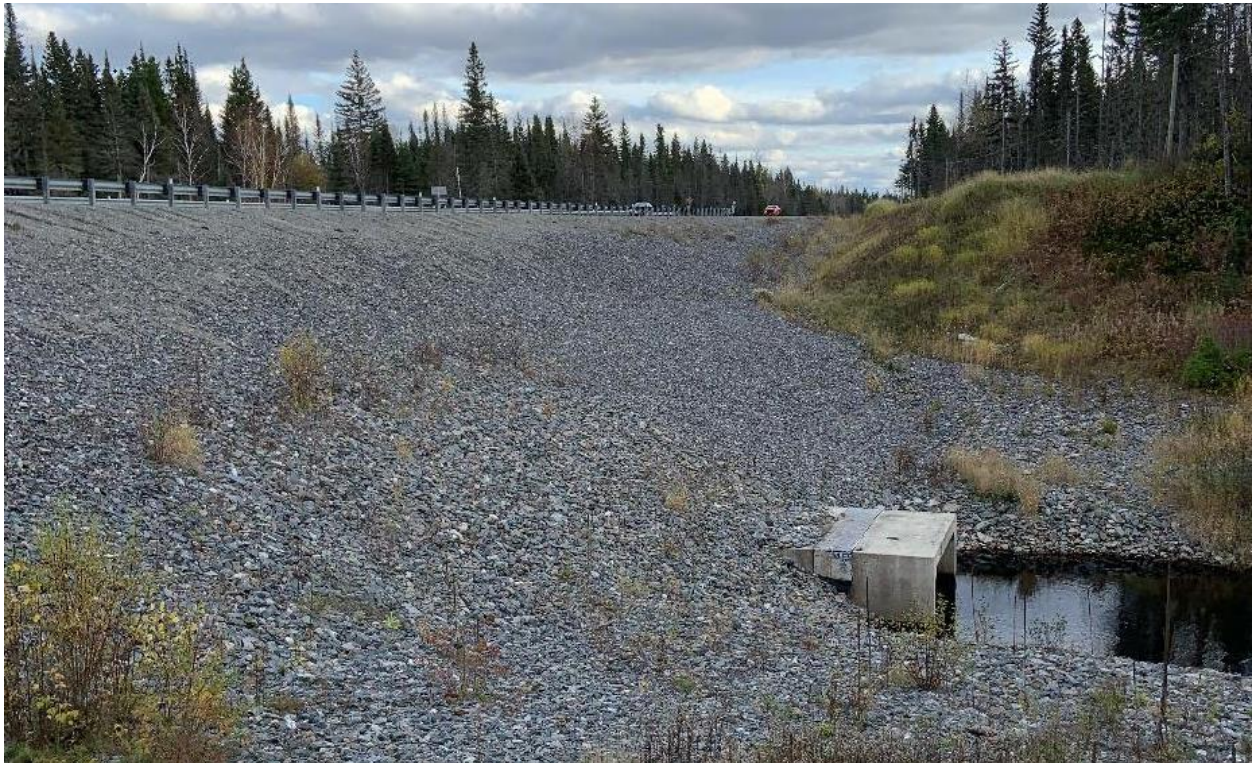
Photo 7: Erosion armouring/protection on fill slope to Jocko Creek
