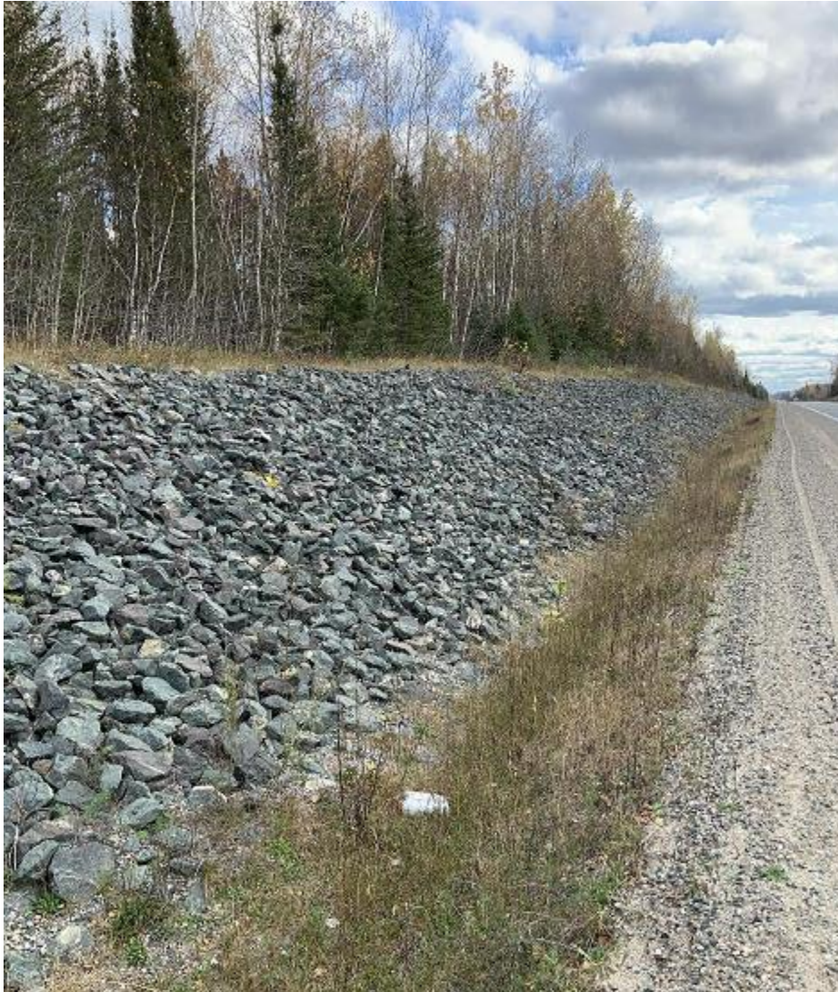
Photo 6: Erosion armouring/protection on cut slope along Highway 655.
