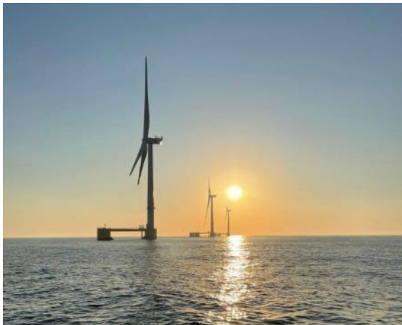
Figure 3: WindFloat Atlantic Semi-Submersible Floating Offshore Wind Farm, Portugal.
