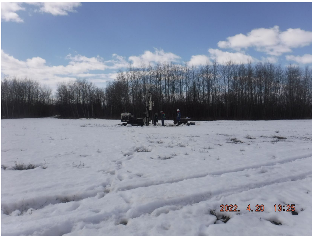
Photograph 2: Looking west towards BH22-2 (WTP Location)
