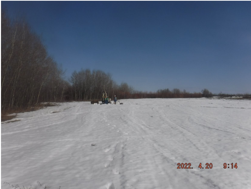
Photograph 1: Looking north towards BH22-1 (SPS Location)
