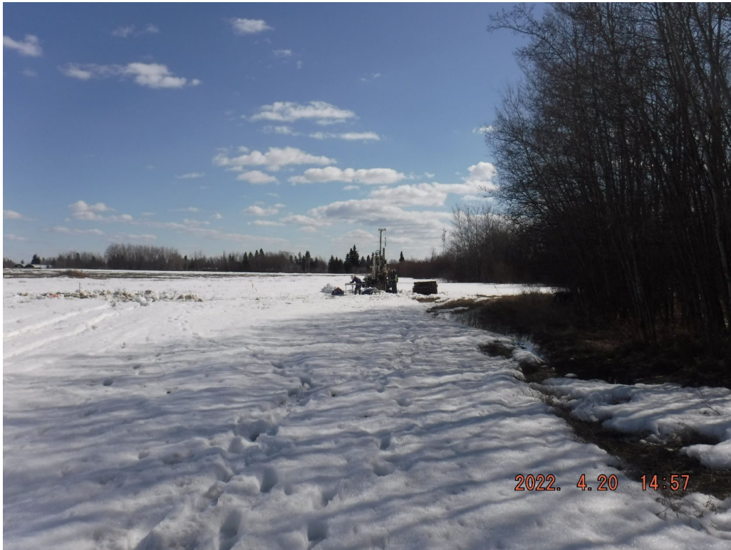
Photograph 3: Looking south towards BH22-3 (WTP Location)
