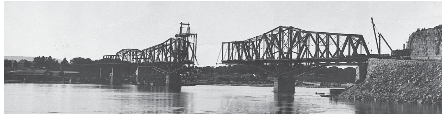
The Interprovincial Bridge (now Alexandra Bridge) during construction, 1901. Source: LAC/Topley/PA-013866
