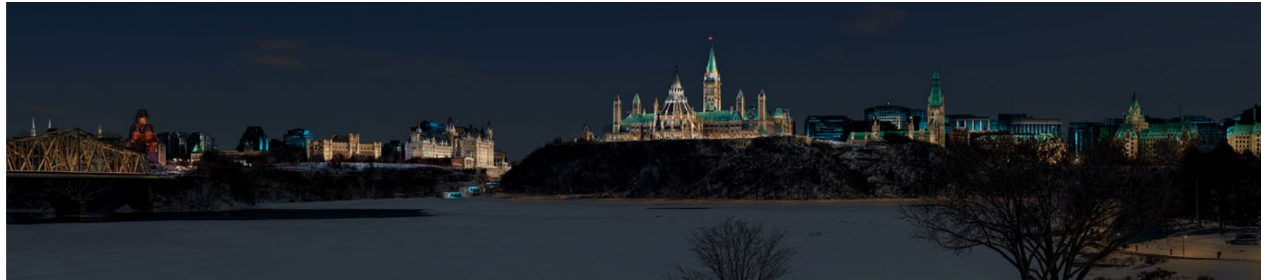
Example of adequate lighting scheme. Source: Capital Illumination Plan
