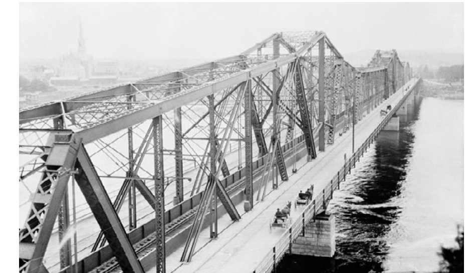
Historical images of Alexandra Bridge. Source: NCC
