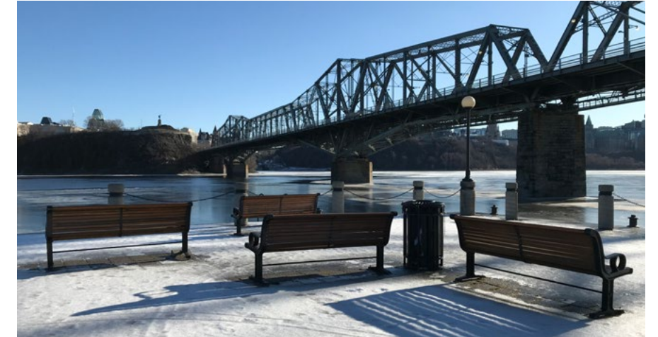
Seating area by Alexandra Bridge Source: Alexandra Bridge Replacement Program and Design guidelines
