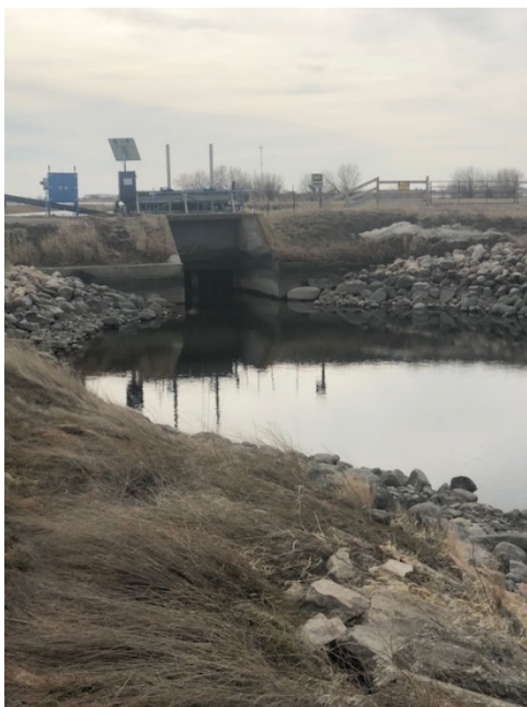
Photo 1 Phase 1- Taber Lake Outlet Structure
