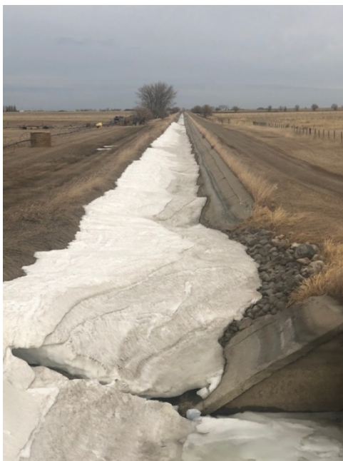
Photo 2 Phase 1 – Beginning of Channel Drain looking west
