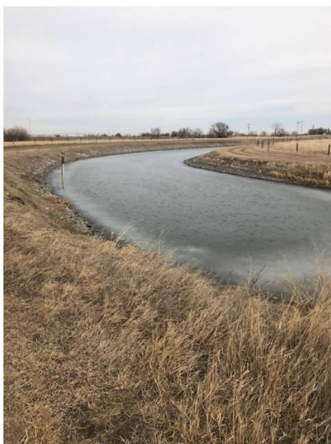
Photo 5 Phase 2 – Horsefly Outlet channel looking north
