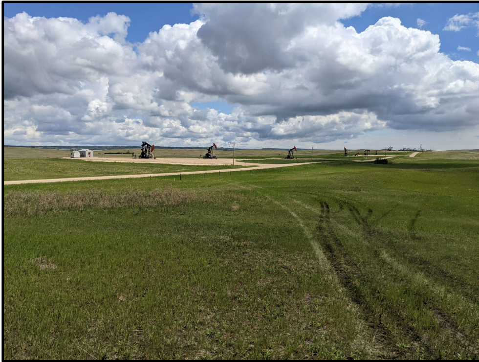
Photograph #1: Northeast view from site location
