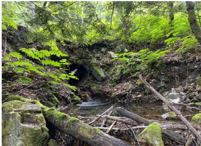
Photo 3 - Culvert outlet at Haisla Blvd.
