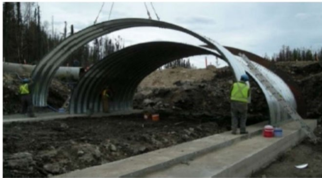
Open Bottom Steel Arch Culvert Under Construction
