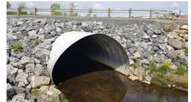
Steel Arch Culvert
