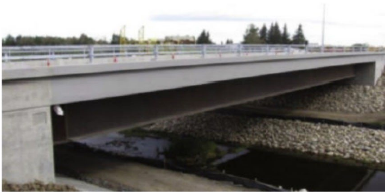
Typical bridge proposed for WSR
