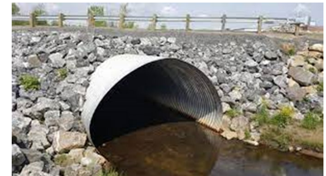
Steel Arch Culvert
