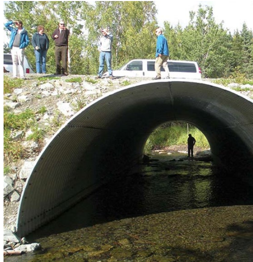
Open Bottom Steel Arch Culvert In Service
