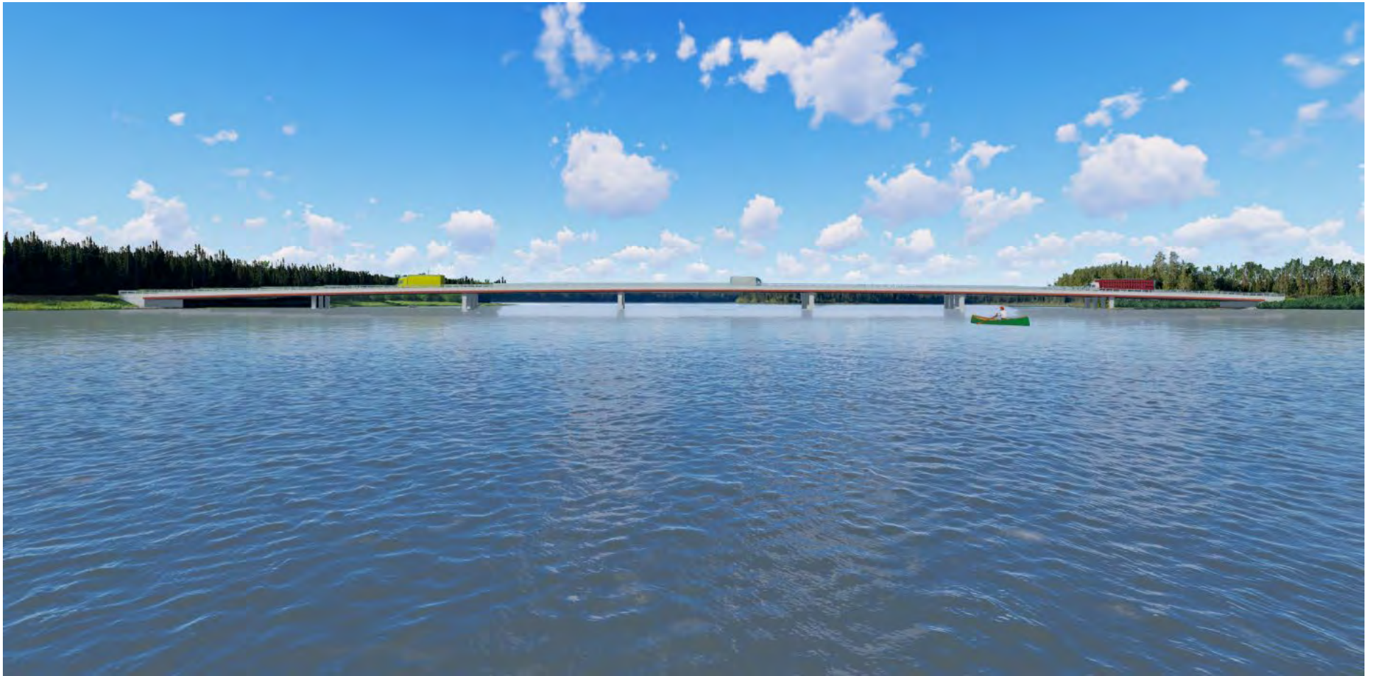
Figure 7.2: Winisk Lake Crossing – Post-Construction – Viewing South
