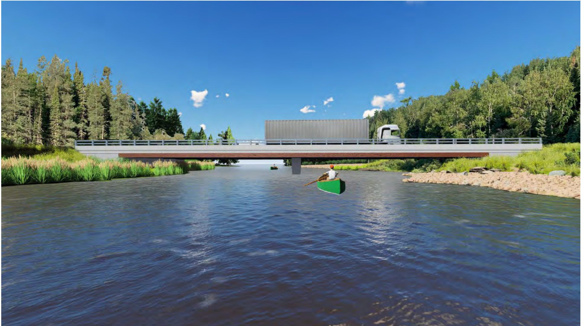
Figure 7.6: Winiskisis Channel Crossing – Post-Construction – Viewing West
