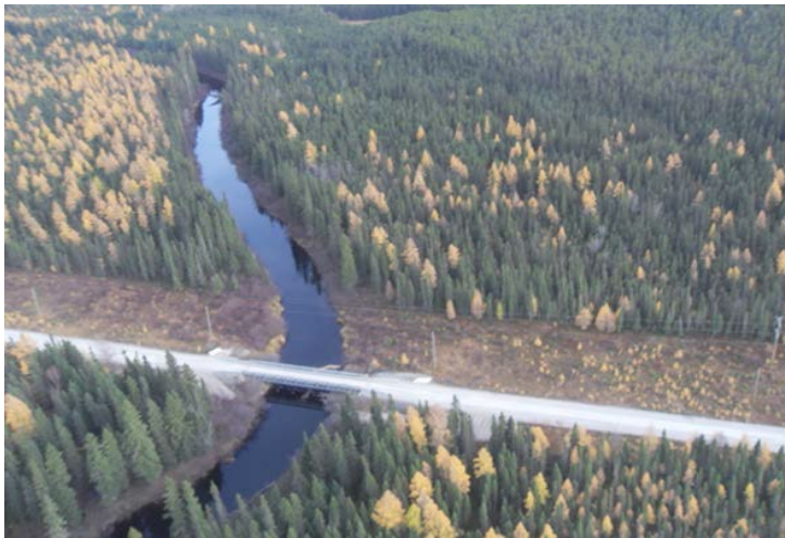
Figure 2.2: Example of Single-span Major Watercourse Crossing Structure
