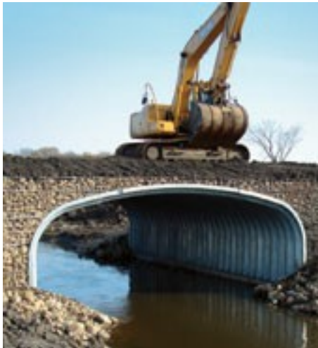
Figure 2.1: Example of Minor Watercourse Crossing Structure (Culvert)
