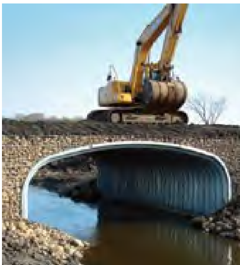
Figure 2.1: Example of Minor Watercourse Crossing Structure (Culvert)
