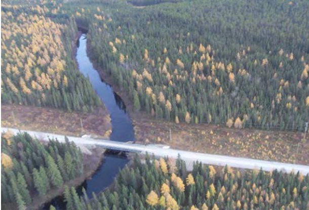
Figure 2: Example of Single-span Major Watercourse Crossing Structure
