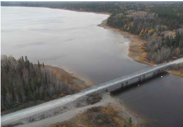
Figure 3: Example of Multi-span Major Watercourse Crossing Structure
