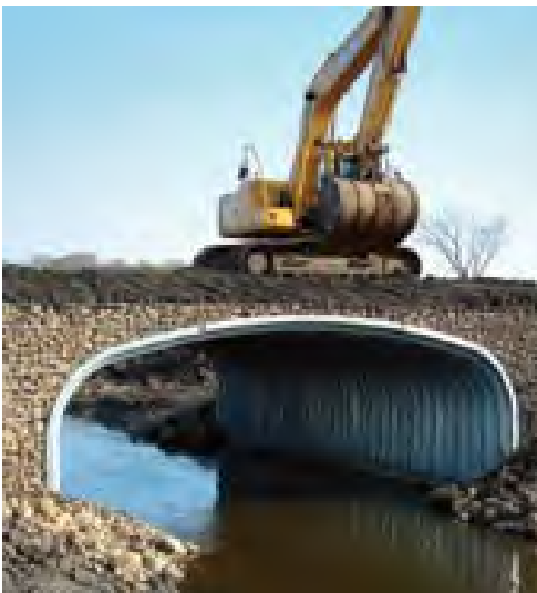
Figure 1: Example of Minor Watercourse Crossing Structure (Culvert)
