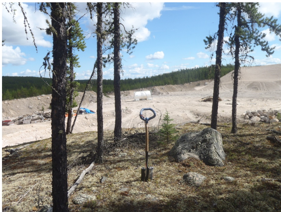
Photo 7: View of existing gravel pit intersected by Phoenix 3 access road option, looking northeast.
