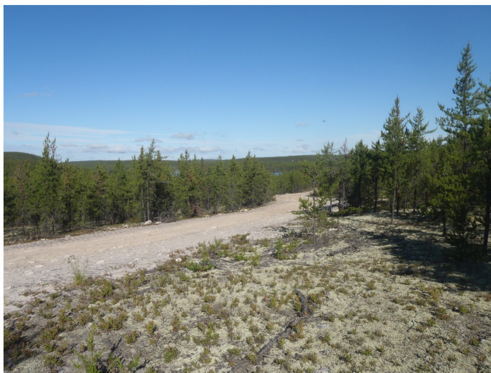
Photo 6: View of existing road within Phoenix 3 access road option, looking northwest.
