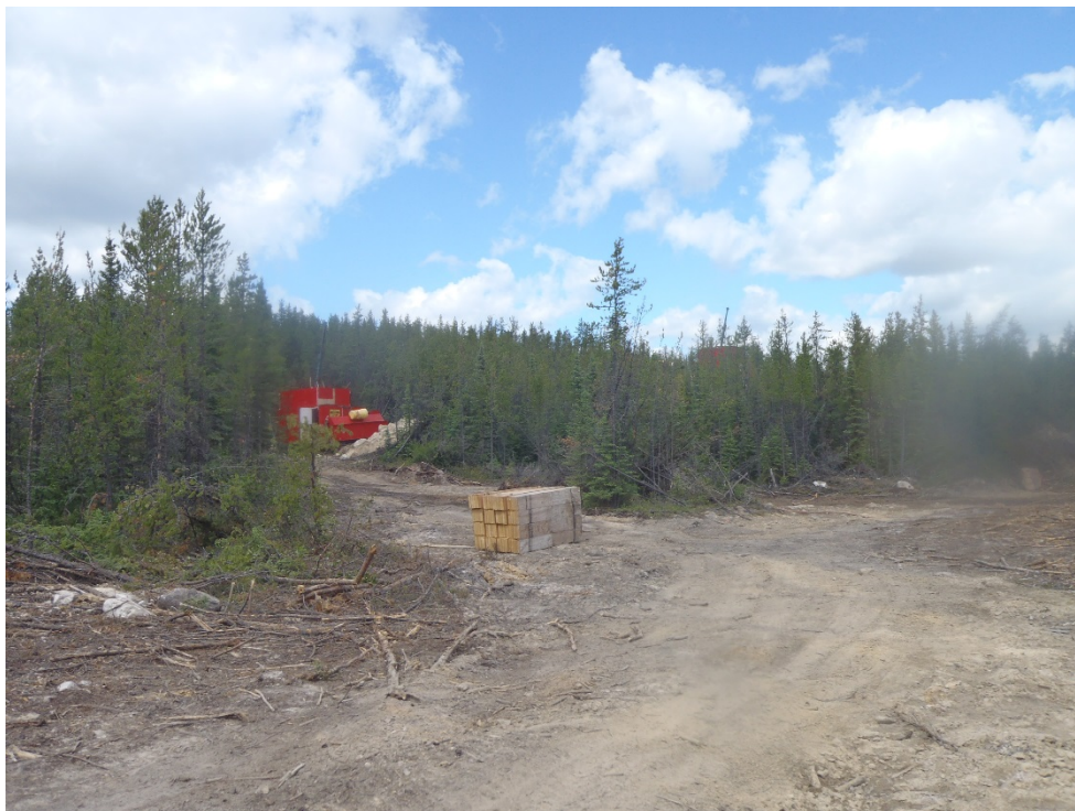
Photo 13: View of drilling activities at Gryphon infrastructure site, looking north.
