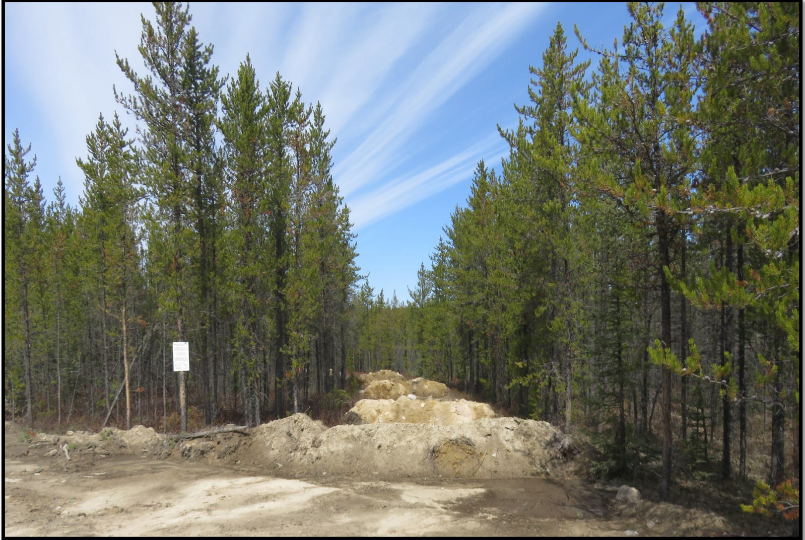
Photograph 4. Status of trench & pile treatment May 2022.
