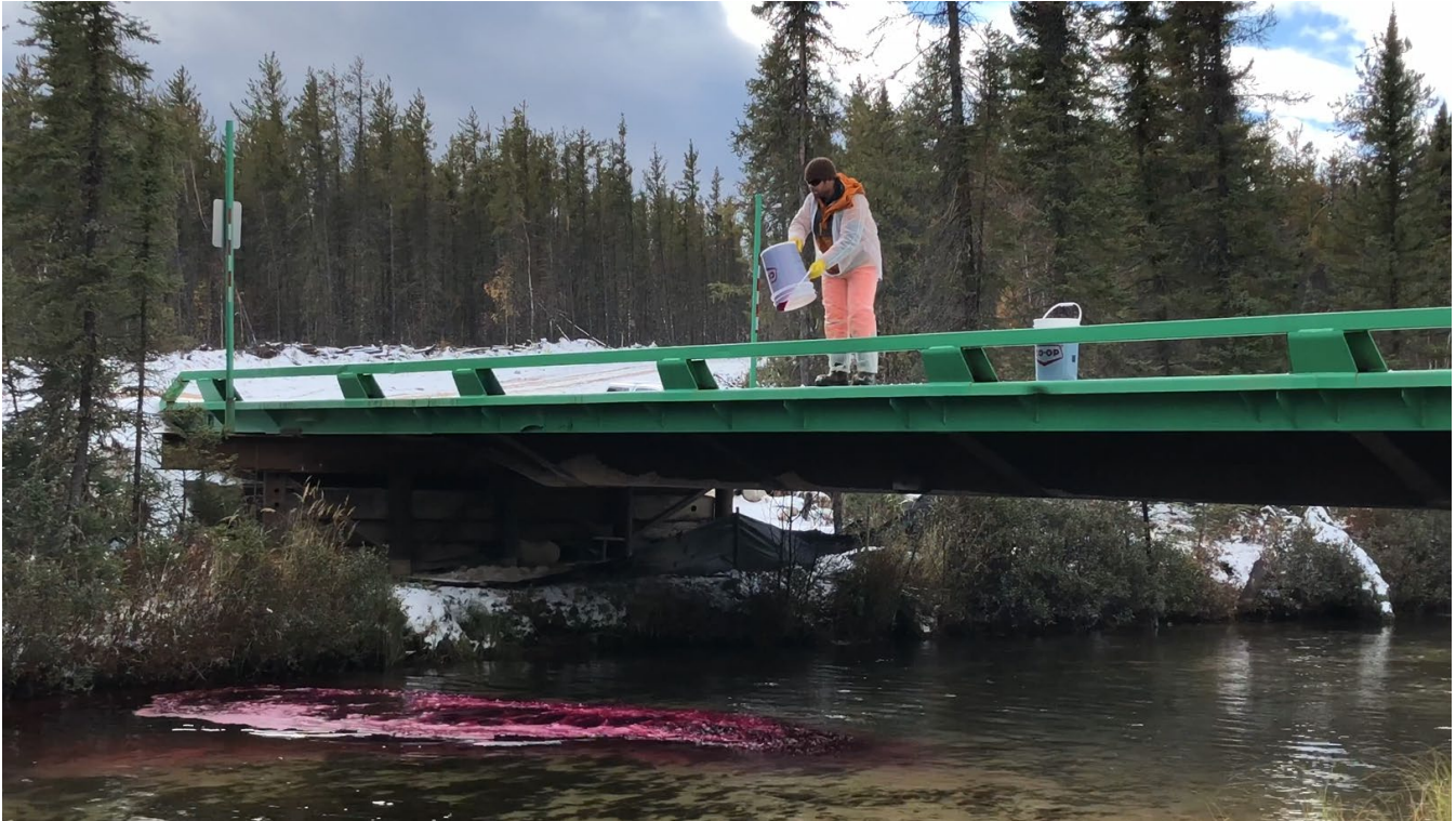
Figure 7: Dye Release from the Access Road Bridge, 30 September 2018 at 13:51
