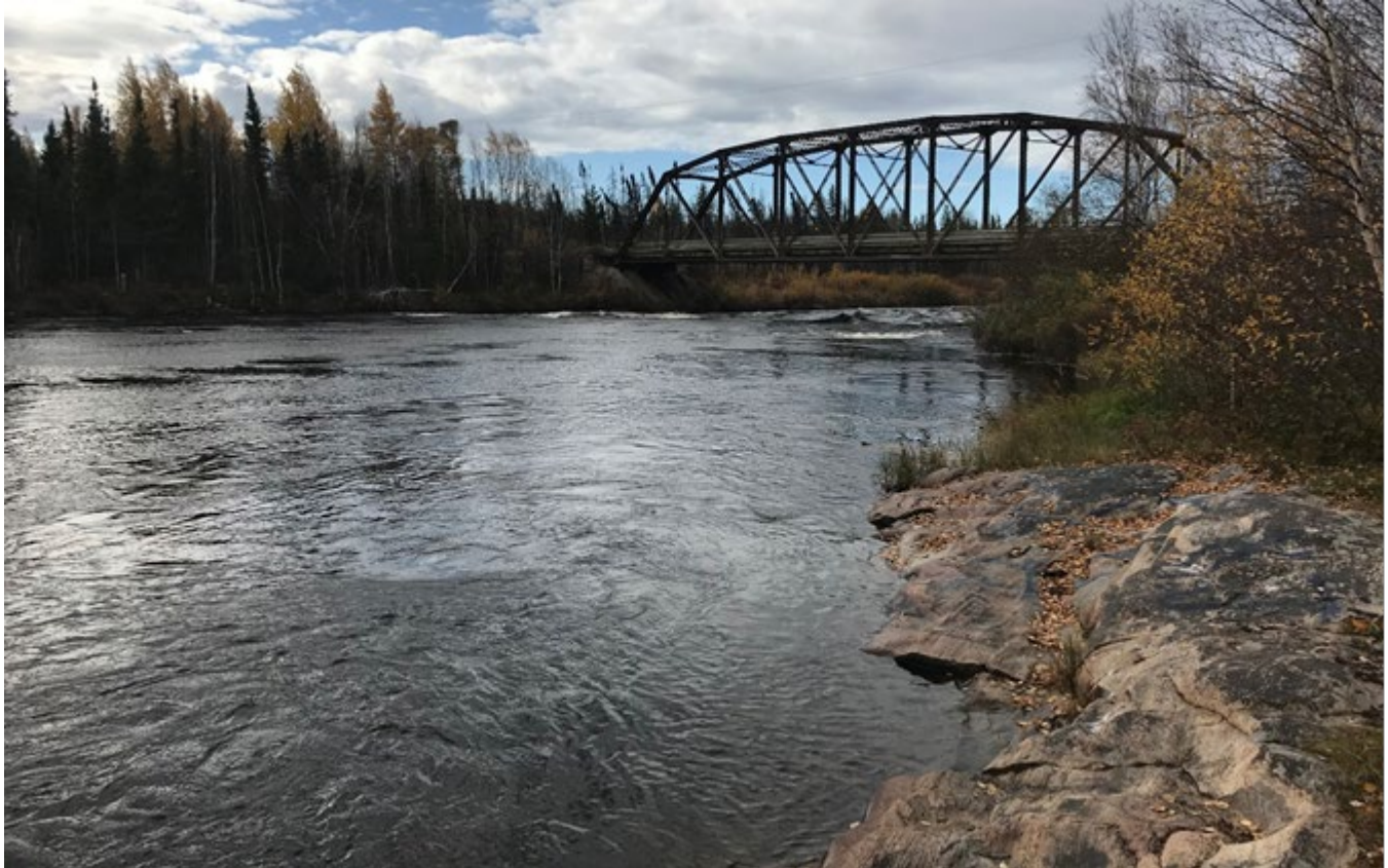
Figure 37: Clearwater River at Warner Rapids, CR-WC-MS-09
