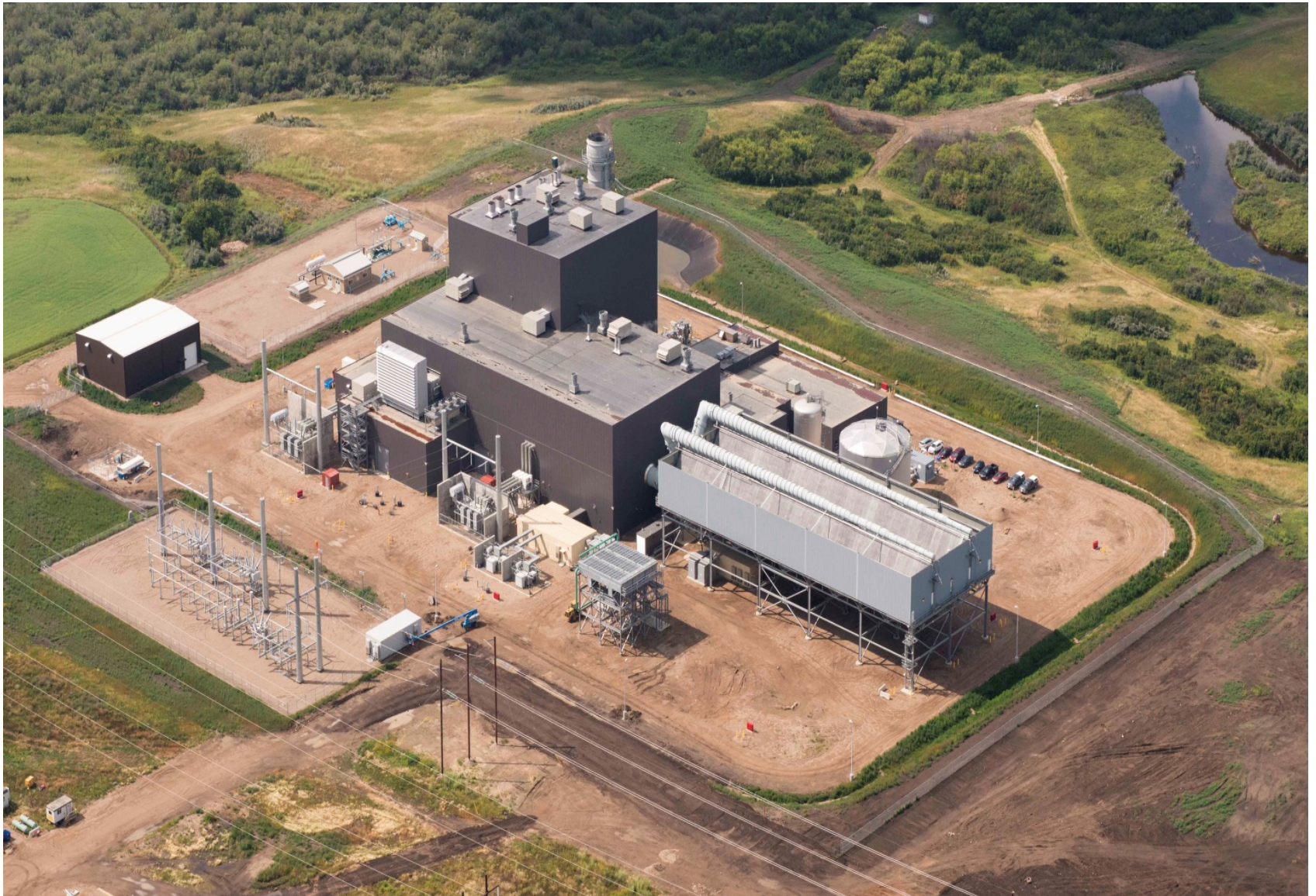
North Battleford Generating Station - Combined Cycle Power Plant, 2013 16
