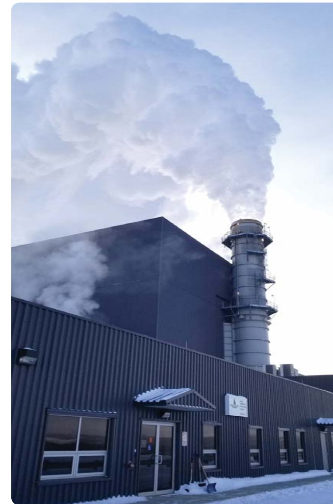
Like your furnace chimney in winter, there is a steady steam plume consisting of mostly water vapour. This photo was taken at the North Battleford Generating Station on a cold day in February.
