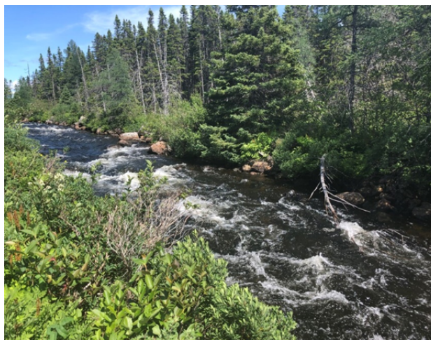
Photo 8 North Twin Brook Outlet Constructed Channel
