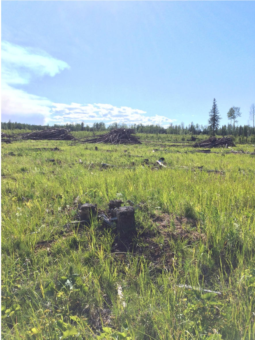
Figure 5-5 Cascade Power Plant, Site Photo Showing Vegetation Clearing
