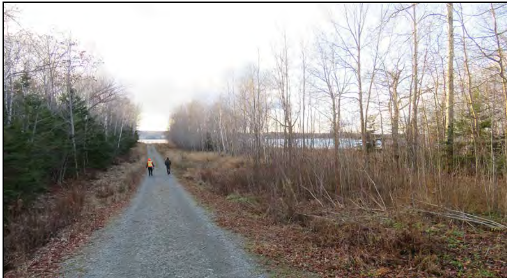
PLATE 2 Pipeline Corridor at Indian Cross Point, facing west toward the East River of Pictou. December 7, 2017.
