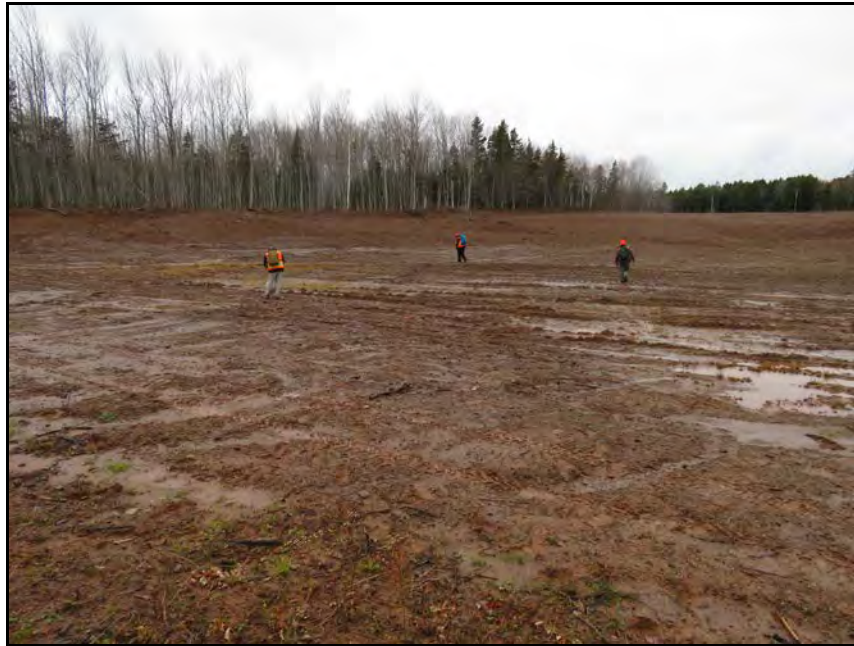
PLATE 29: Reconnaissance within the borrow pit that lies to the southwest of Former Settling Pond 2. Facing southeast. December 4, 2017.
