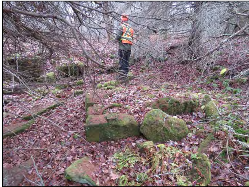
PLATE 19: Chimney base within the house cellar at the Donald McArthur Site. Facing east. December 5, 2017.
