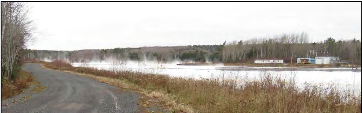
PLATE 4 Aeration Stabilizing Basin (centre) and Electrical Building (right). Facing northwest. December 5, 2017.
