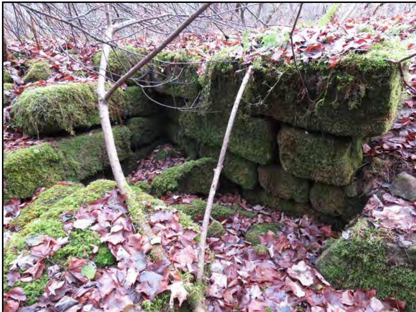
PLATE 18: Northeast corner of the Donald McArthur house foundation. Facing northeast. December 5, 2017.
