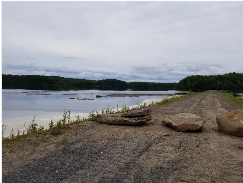
Photo 9: Berm (WC1) in stabilization lagoon (1 of 4), July 25, 2019
