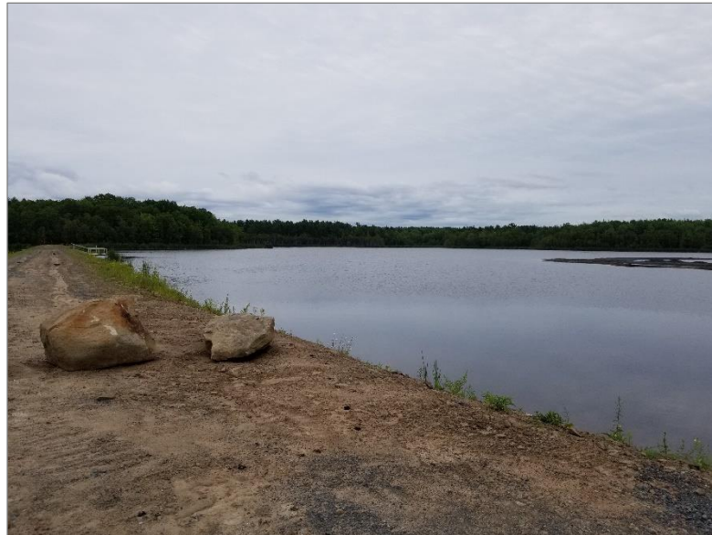
Photo 11: Berm in stabilization lagoon (3 of 4), July 25, 2019
