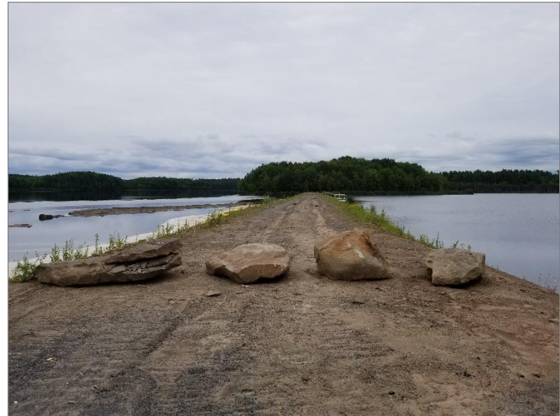
Photo 10: Berm in stabilization lagoon (2 of 4), July 25, 2019
